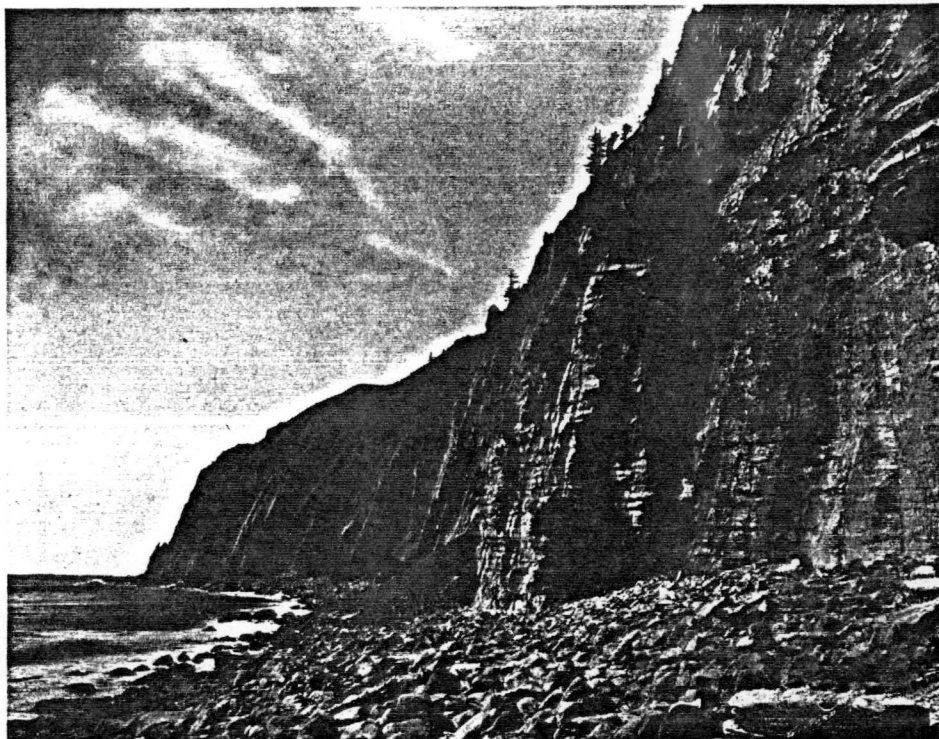
As far north as it is possible to travel, one encounters the bottom of monster slides that have dug their great paths out of the heart of the mountain. (NOTE.—In the center foreground is the foot of Rock Canyon, above which the bridge is being built.)
