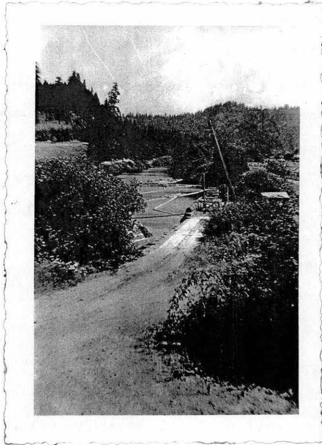
Figure 65. A splash dam site on Daniels Creek, southeast of the confluence of the Coos and Millicoma Rivers, on the South Fork Branch. A full boom has been taken out recently and new boom guides have been left by the tug. As the logs are dumped into the dam they will be maneuvered about to make a compact raft; the completed boom will be hauled downriver with the tide, to the mill.
