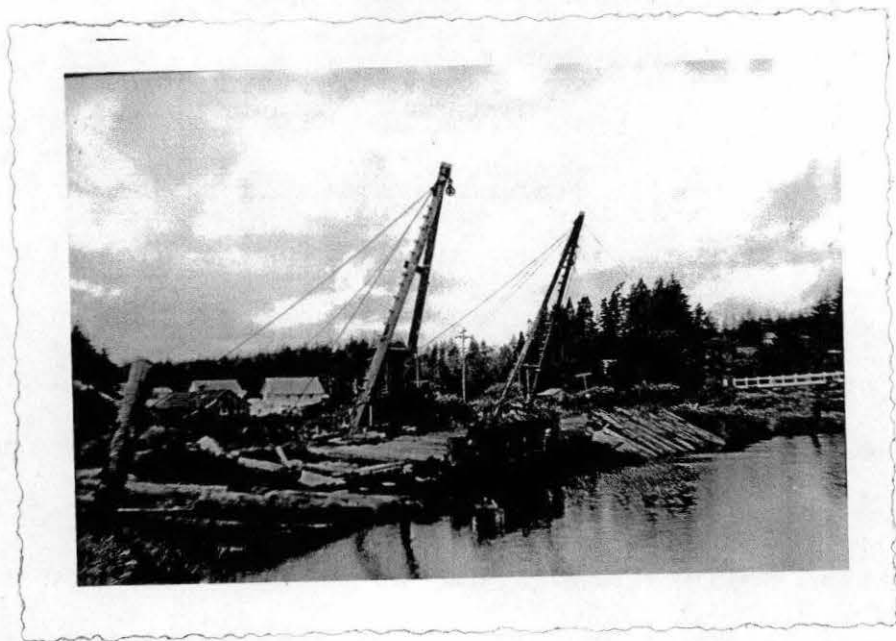
Figure 60. A splash dam and unloading site at Hauser: Hauser in the center background, the Howard bogs to the left, and U. S. 101 passing over the bridge to the right. A site much like this is used by the Pulp Company to raft up their logs from Lake Tahkenitch.
