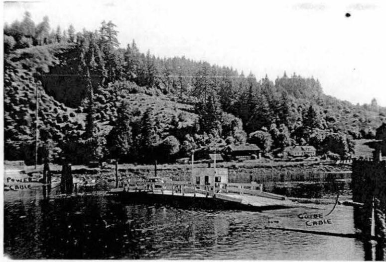
Figure 84. The Enegren Ferry crossing the Coos River from south to north. The power unit is housed in the control house in the middle of the ferry, with two winch lines to provide the means of movement. The cable extending out to the front takes the strain of the motor pulling, while that to the rear acts to control the direction.
