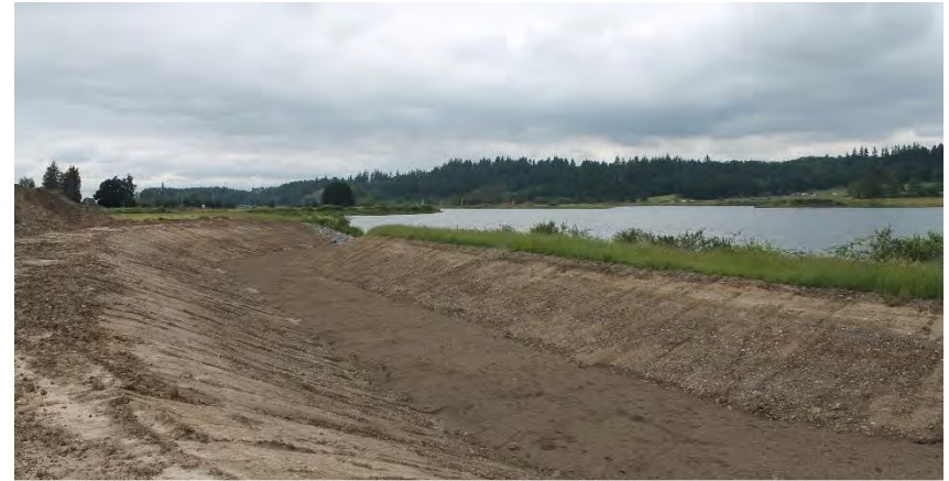
Large swale constructed to manage runoff on site, June 2017
