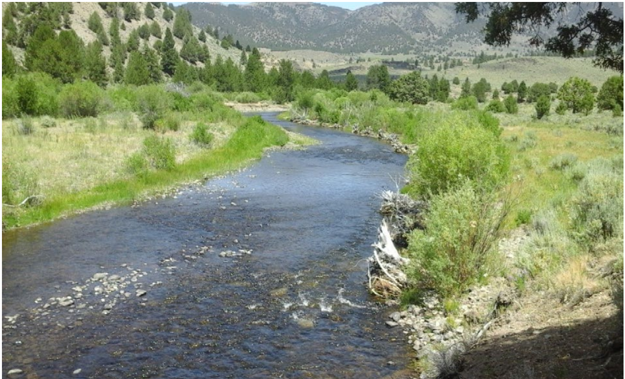
Figure 5.8 Strohm streambank stabilization and riparian restoration site in 2020.
