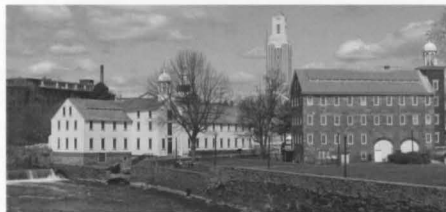
Rehabilitated factory buildings in the Blackstone River National Heritage Area. Image Courtesy of MassMoments.Org
