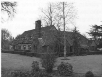
Oregon State Forester's Office Building, Salem, constructed 1938. Photo by author.
