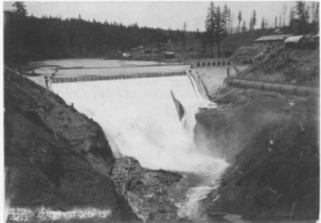
The Condit Dam in the Spring of 1913. Image courtesy of the Columbian.
