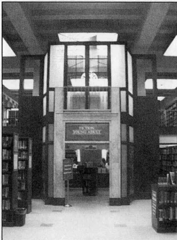
Illustration 3-28 Portal Created in 1986 Rehabilitation, Flathman, 2007
