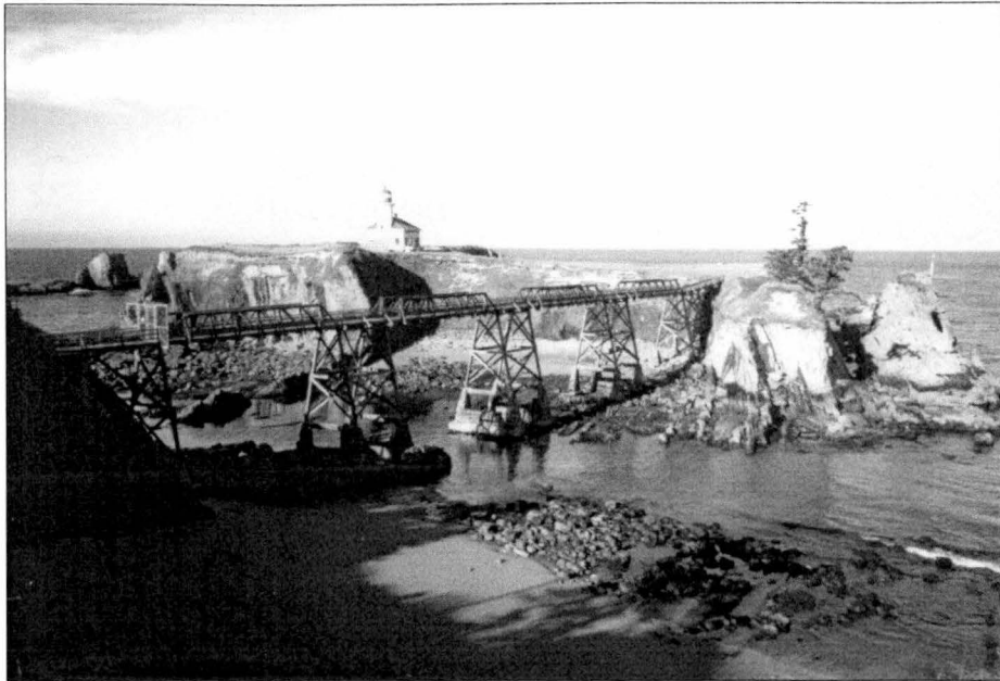
Figure 49. Bridge to Lighthouse Island, 1999. Source: Author.
