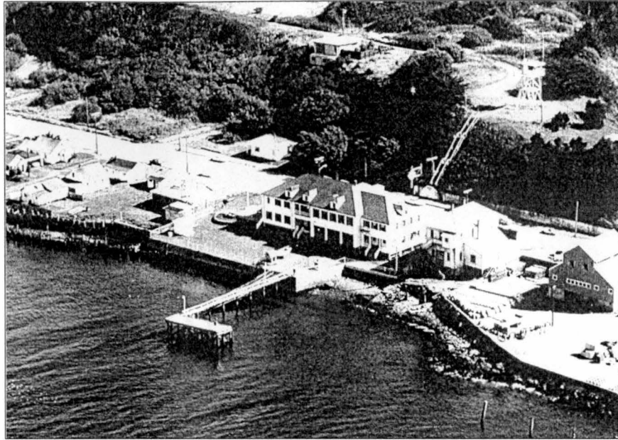
Figure 101. Aerial of Station with Current Coast Guard Lookout at Upper Right and "Little America" to Left, 1966. Source: National Archives (RG 25-CGS, Box 2, Folder Coquille River Station).
