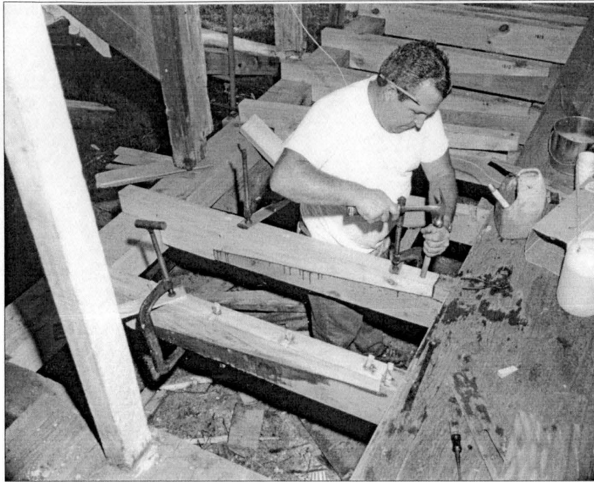
Figure 182. Splicing Floor Joists at Block Island Life-Saving Station, Rhode Island, 1970. Source: Mystic Seaport (#70-8-364).
