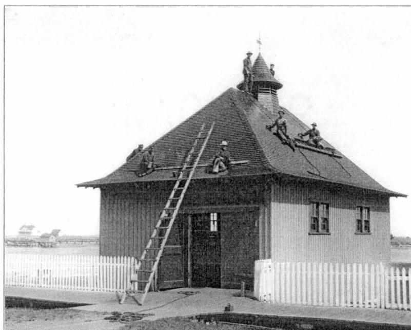
Figure 181. Surfmen Painting the Boathouse Roof, Coquille River Life-Saving Station, Circa 1900. Source: Bandon Historical Society.
