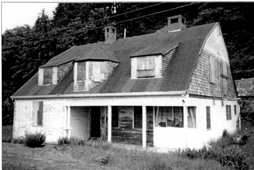
Figure 157. Station House (1907), Tillamook Bay Life-Saving Station, 1997. Source: Author.
