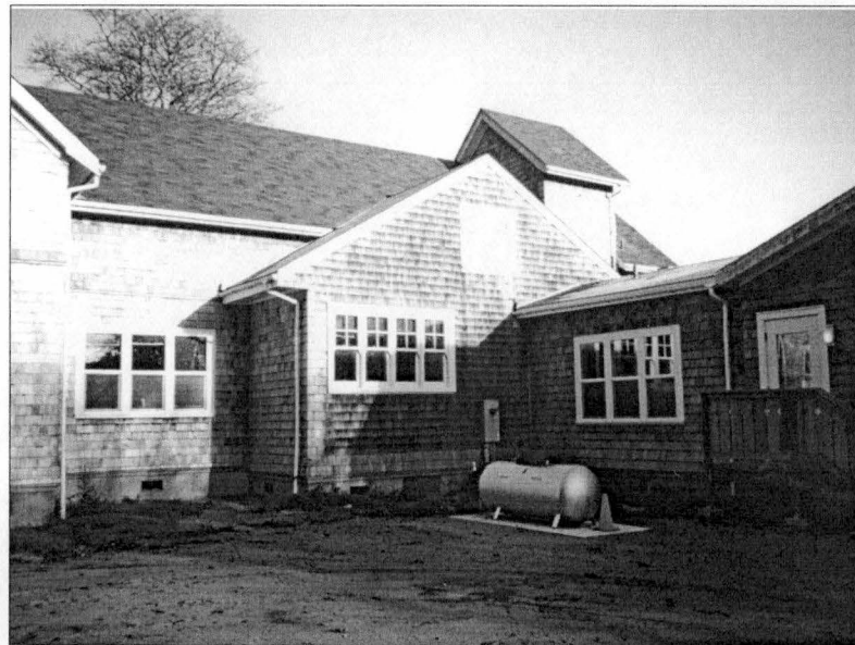
Figure 190. Keeper's Dwelling (1915) Enveloped, Coos Bay Lifeboat Station, 1999. Source: Author.
