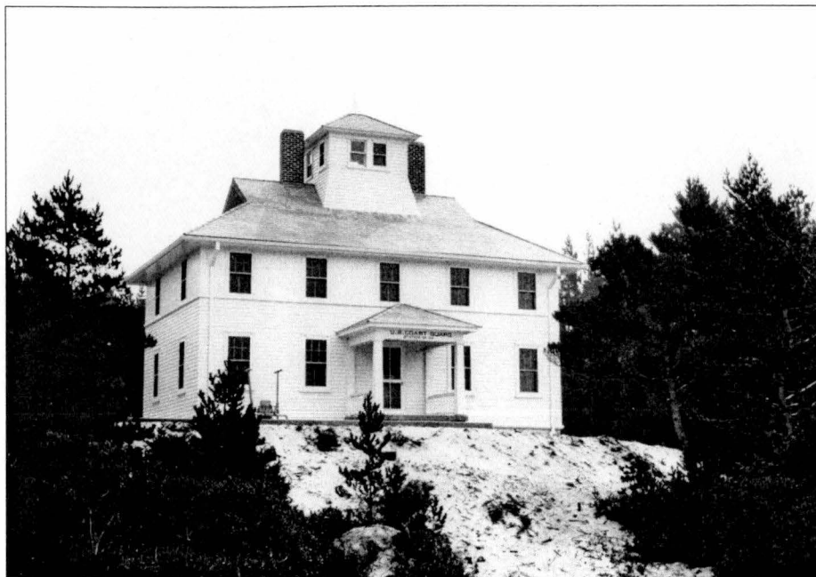
Figure 162. Siuslaw River Lifeboat Station, 1917. Source: U.S. Coast Guard Headquarters (Siuslaw River File).
