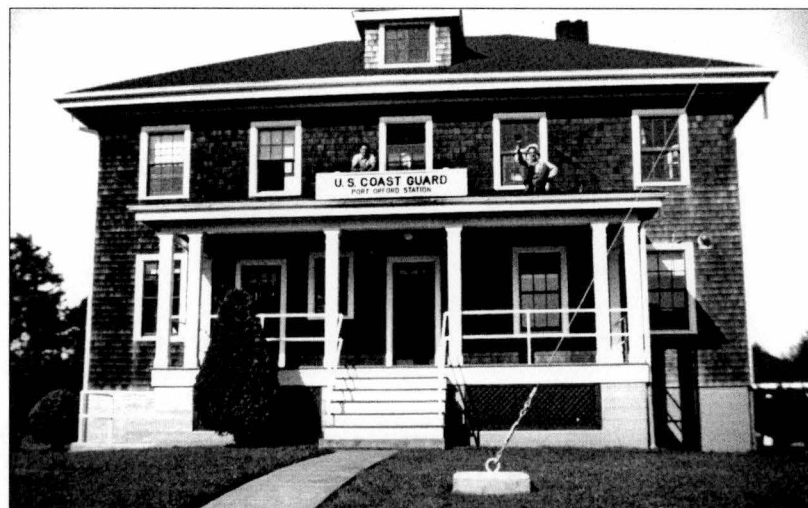
Figure 174. Station House, Port Orford Lifeboat Station, Circa 1940. Source: Oregon State Historic Preservation Office (Port Orford File).
