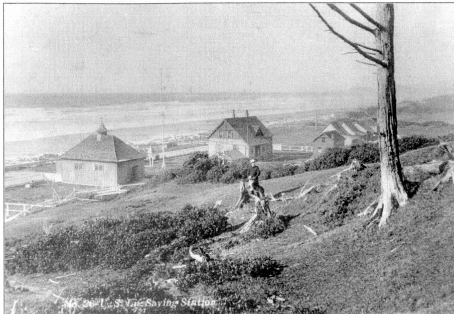
Figure 120. South Beach Station, 1906. Source: Lincoln County Historical Society (LCHS #590).
