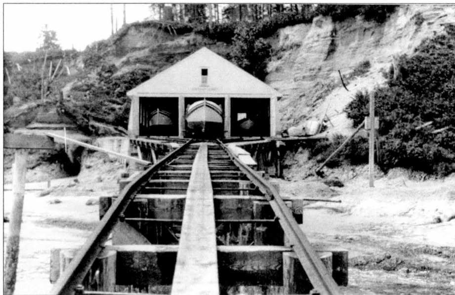
Figure 65. Coos Bay Lifeboat Station, Boathouse Ramp, 1923. Source: U.S. Coast Guard Headquarters (Coos Bay File).
