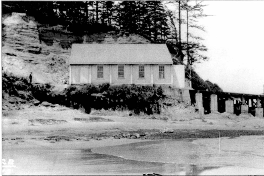
Figure 64. Coos Bay Lifeboat Station, Boathouse, 1923. Source: U.S. Coast Guard Headquarters (Coos Bay File).
