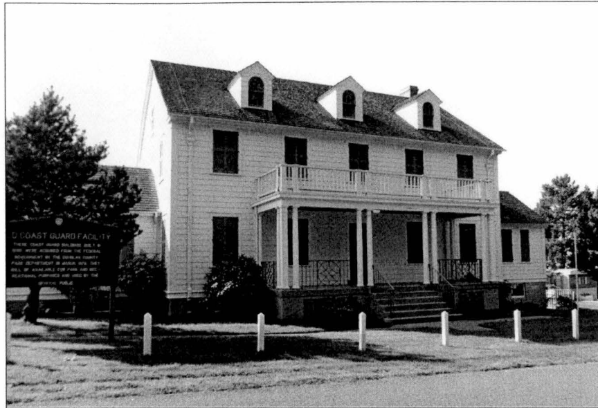
Figure 116. Station House at Umpqua River Lifeboat Station, 1991. Source: Oregon State Historic Preservation Office (Umpqua River Coast Guard Station File).
