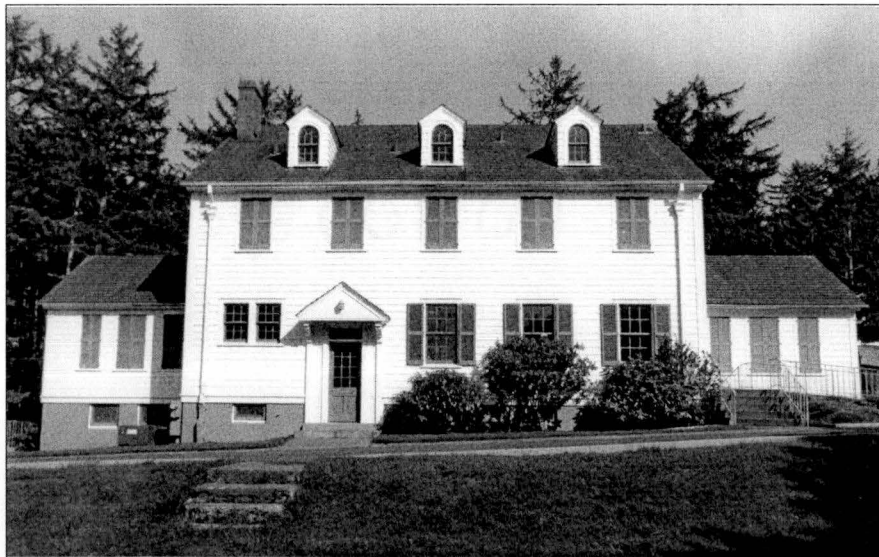
Figure 117. Rear Elevation of the Station House at Umpqua River, 1991. Source: Oregon State Historic Preservation Office (Umpqua River Coast Guard Station File).
