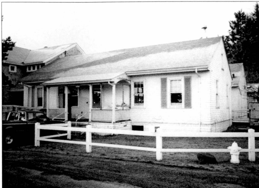
Figure 70. Former Crew's Dwelling (1915), Coos Bay Lifeboat Station, 1999. Source: Author.
