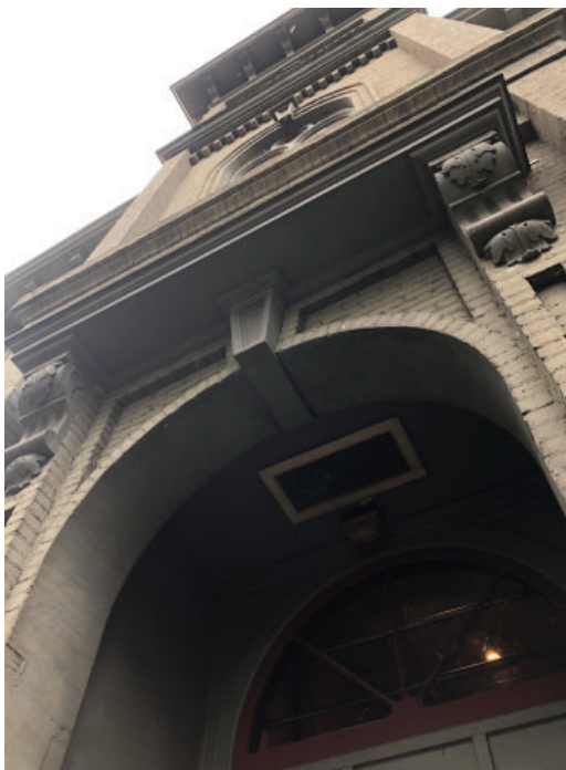
Air vent and exterior light above East entrance, not original
