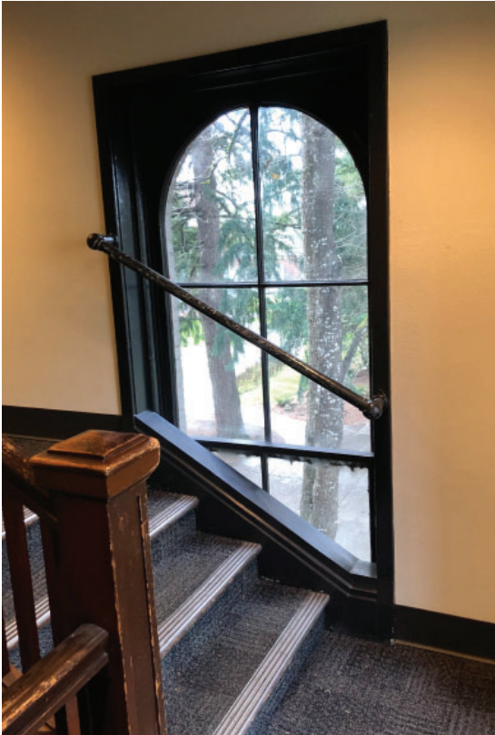
First Floor Stairwell. Windows were split between two floors in major stairwells following the addition of mezzanine levels.
