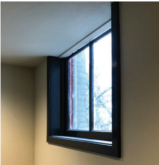
Window in mezzanine level 1 hallway
