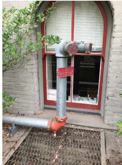
Exterior fire utility connection added along north elevation
