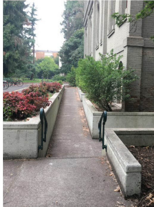
Original stairs removed, ramp added to create an ADA entrance
