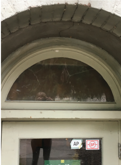
Door and original window trims were painted
