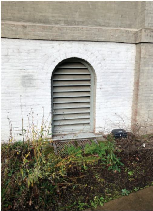
Original window infilled to create basement ventilation
