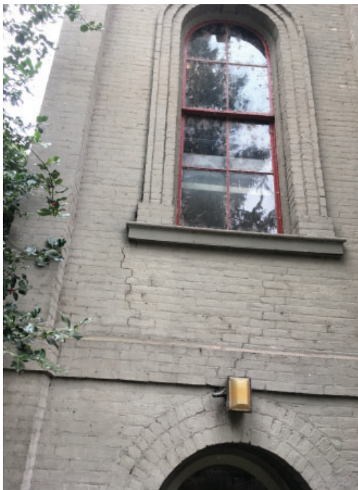
Original wood window trims were painted, light fixtures added
