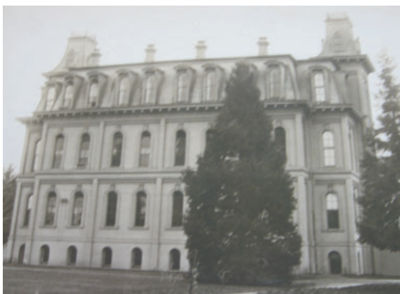
University Hall South Facade, 1876
