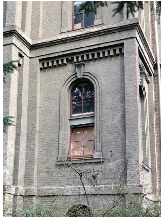
Window sills were painted from original color
