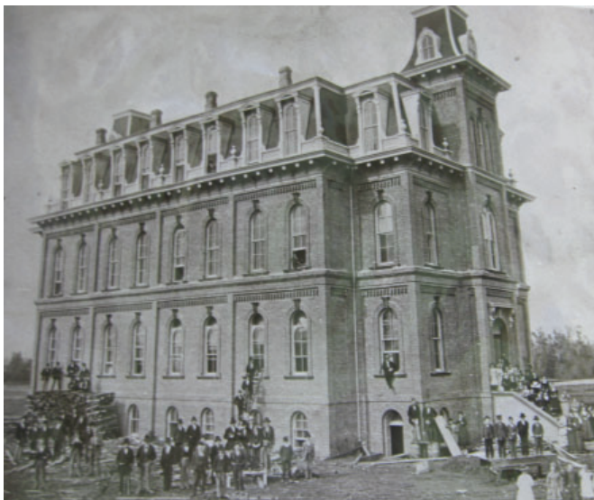
University Hall North Facade, Inception Era
