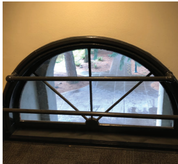
First Floor Stairwell. Bars added over split level windows.
