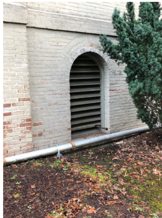
Basement window infilled, used for ventilation
