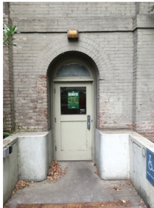
ADA entrance through basement level located at northwest corner, incompatible light fixture
