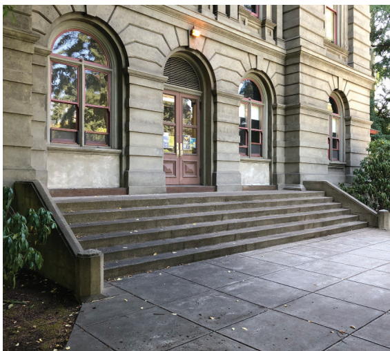
Windows on either side of the entrance were originally doors. Glass panels may have been added to the central wooden door, or it may be an entirely different door (further research needed).
