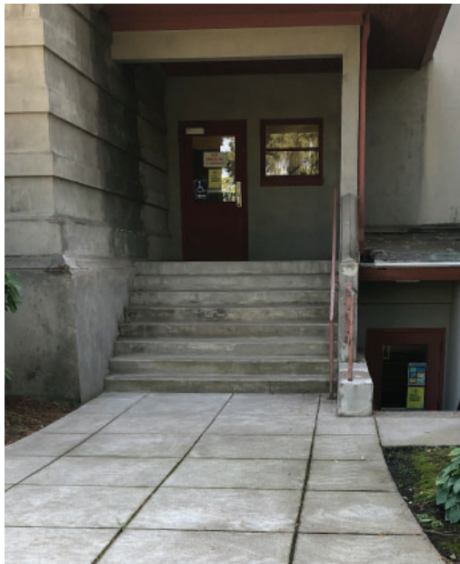
Stairs added during Robinson Theater addition.
