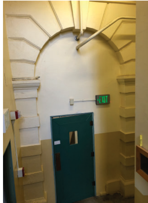
West facade as viewed from inside the Robinson Theater (2nd floor stairwell), window infilled to create entrance into Villard Hall, archway preserved and covered in finishing material as to match the interior of the Robinson Theater.
