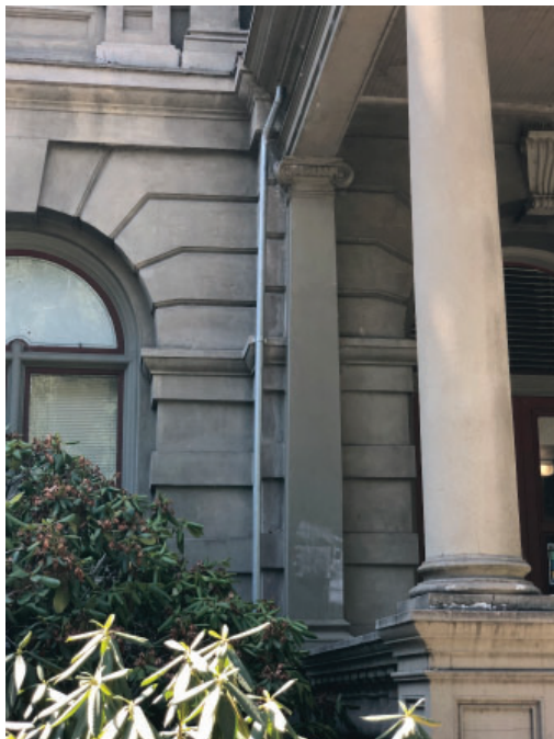
Roof drainage downspout.
