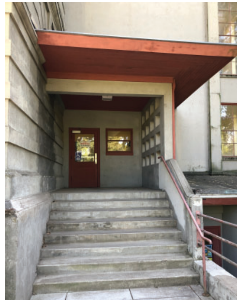
Cover added during Robinson Theater addition, window infilled on Villard Hall.
