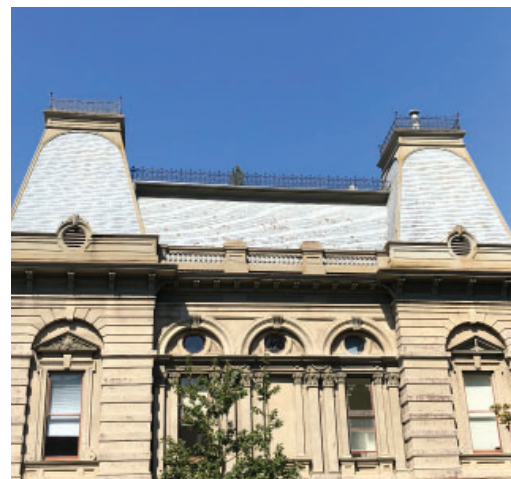
Missing decorative pediment (right), missing decorative urn details, and painted cedar roof shingles to mimic slate (paint is degrading on some more than others; replaced in kind during restoration).
