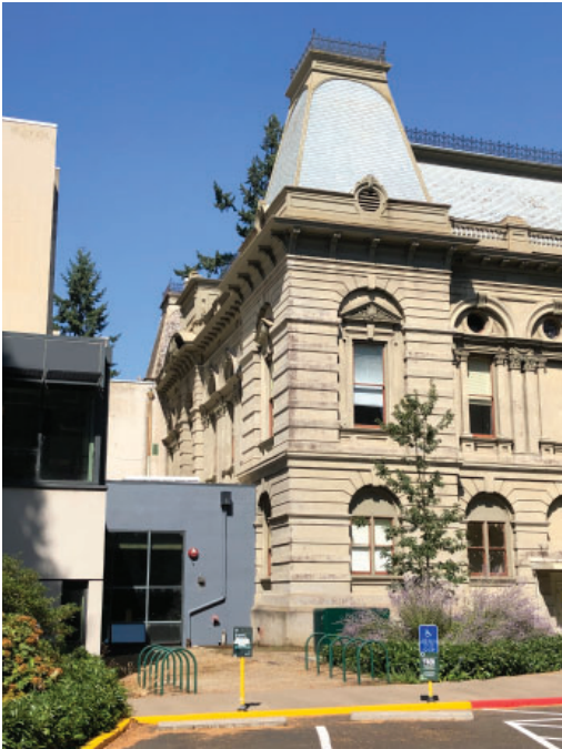
Attachment of the Robinson Theater at West Facade, missing decorative urn details, missing decorative pediment (center), missing exterior center stair and entrance with covered porch and decorative railing and balustrade on roof.
