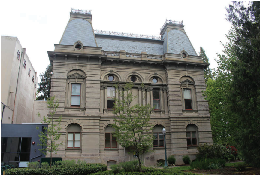
Villard Hall, South Elevation, 2021
