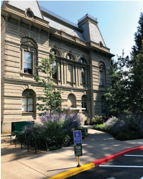
Villard Hall, South Elevation, 2021
