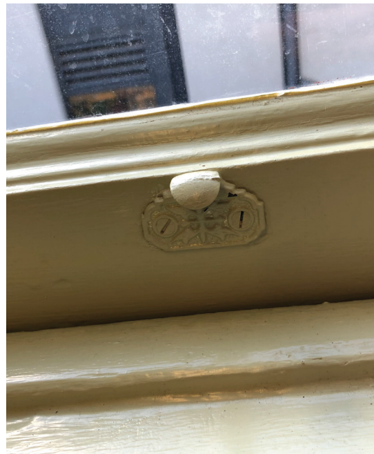
Classroom 201 hardware detail
