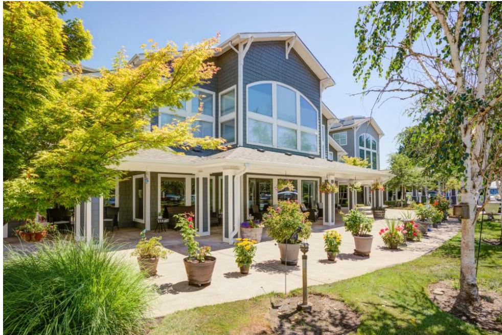
Figure 11. Timber Pointe senior living facility, Springfield, OR
