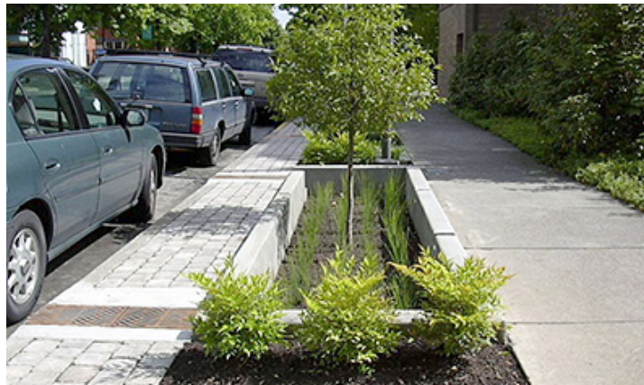
Figure 45: Sidewalk planters for storm water retention.
