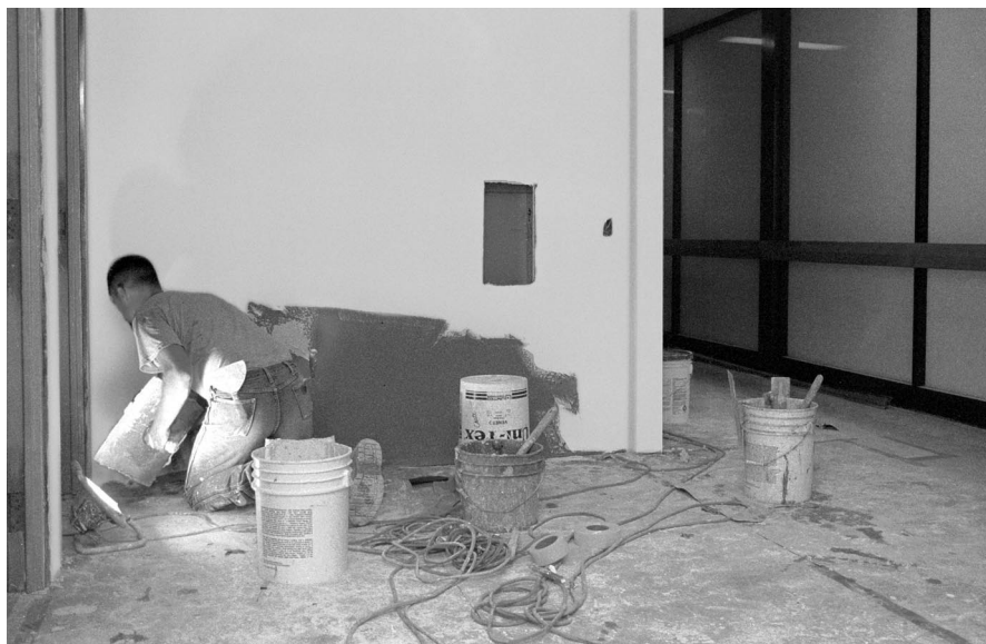
A worker plasters a wall of one of the new Facilities Services offices on the first floor.
