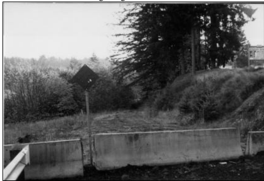
Impacts from 1996 Landslide Event, Dairy Creek Rd. Source: Community Planning Workshop
