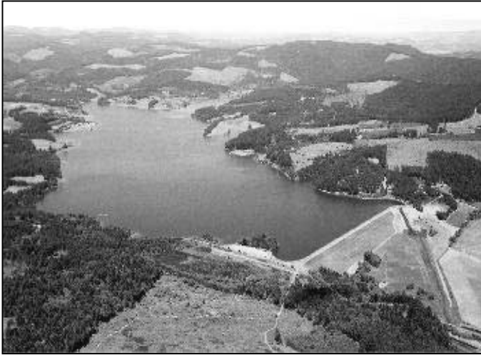
Scoggins Dam Source: Bureau of Reclamation
