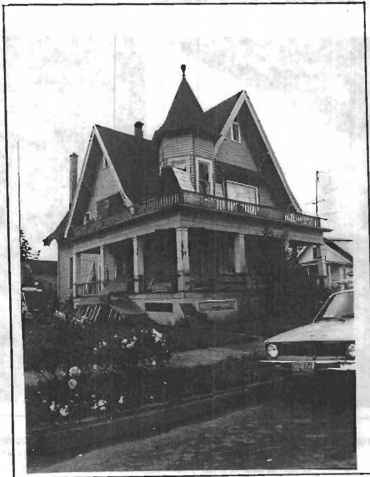
INVESTING IN THE NEIGHBORHOOD: 1910 QUEEN ANNE STYLE HOUSE UNDERGOING RENOVATION
