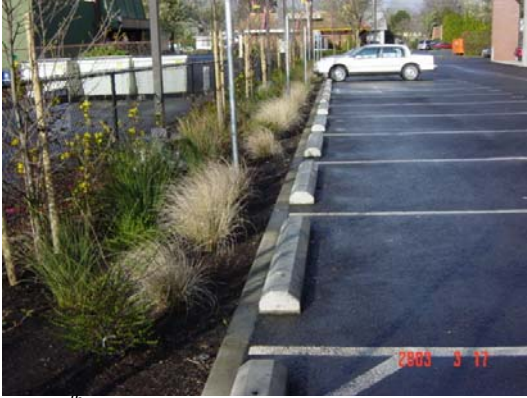
NE 40 th Avenue near Tillamook
