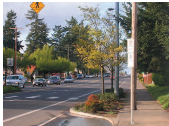
Mid-block curb extension used in conjunction with current pedestrian refuge north of Glisan
