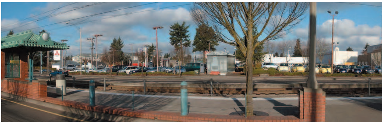
Existing MAX station and auto dealership on Burnside east of 122nd.
