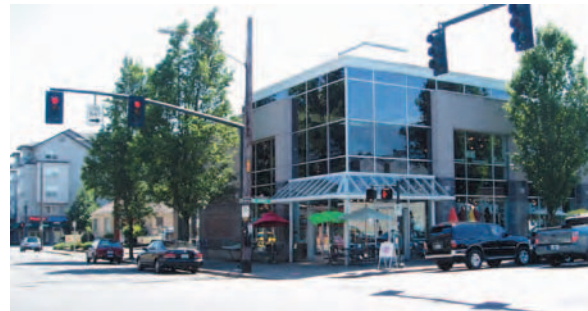
Corner Commercial Development
