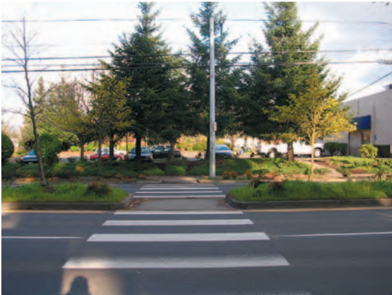
Existing pedestrian refuge island on 122nd north of Glisan
