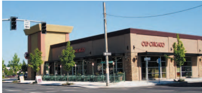
Corner Commercial Development
