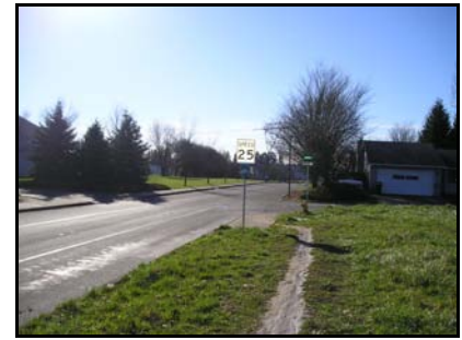
Gaps in the sidewalk hinder pedestrian access to transit.
