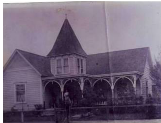
1822 5 th Ave- Miller-Baker House (1899)
