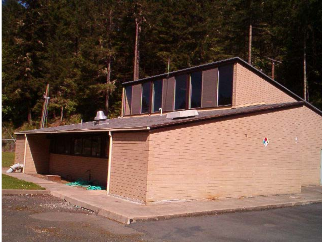
FIGURE 5.3.6 COOPER CREEK WTP BUILDING
