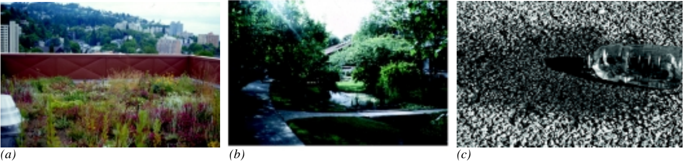
Figure 6.6 Existing examples of green infrastructure storm water mitigation concepts: (a) an eco-roof at the Hamilton Building, Portland, OR; (b) a grass swale in Village Homes, Davis, CA; (c) pervious paving. (photos: CHI)
