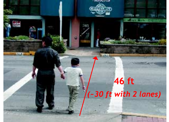
The crosswalk on the north leg of the intersection crosses 3 lanes between shallow curb extensions. The crossing can be shortened by removing a lane and extending the curbs fully.
