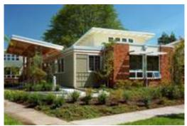
The Moss Street Children's Center operates 32 percent more efficient than code with the help of enhanced mass for passive cooling and night flush, south facing glazing for passive solar gain, radiant floor heating and cooling, and hybrid ground source heat pumps, buried in 300-foot wells.
