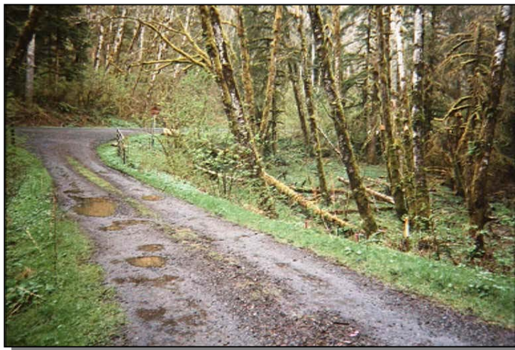
Typical "High clearance" Key Forest road
