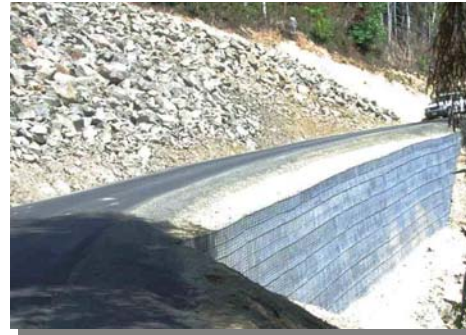
Stabilized mid-slope road
