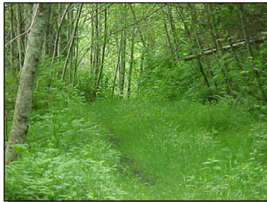
Stabilized, non-Key Forest Road with vegetation encroachment
