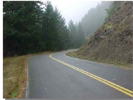
Stabilized mid-slope road
