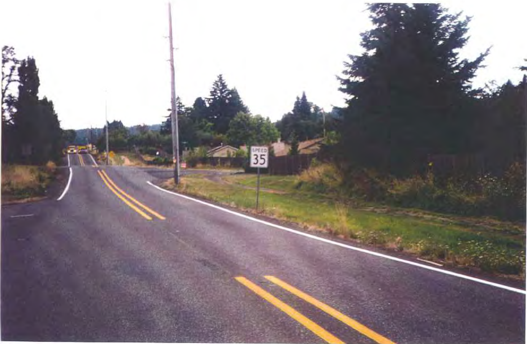
FIGURE A-5 SW 170th Ave. North of SW Bany Rd. - Existing
