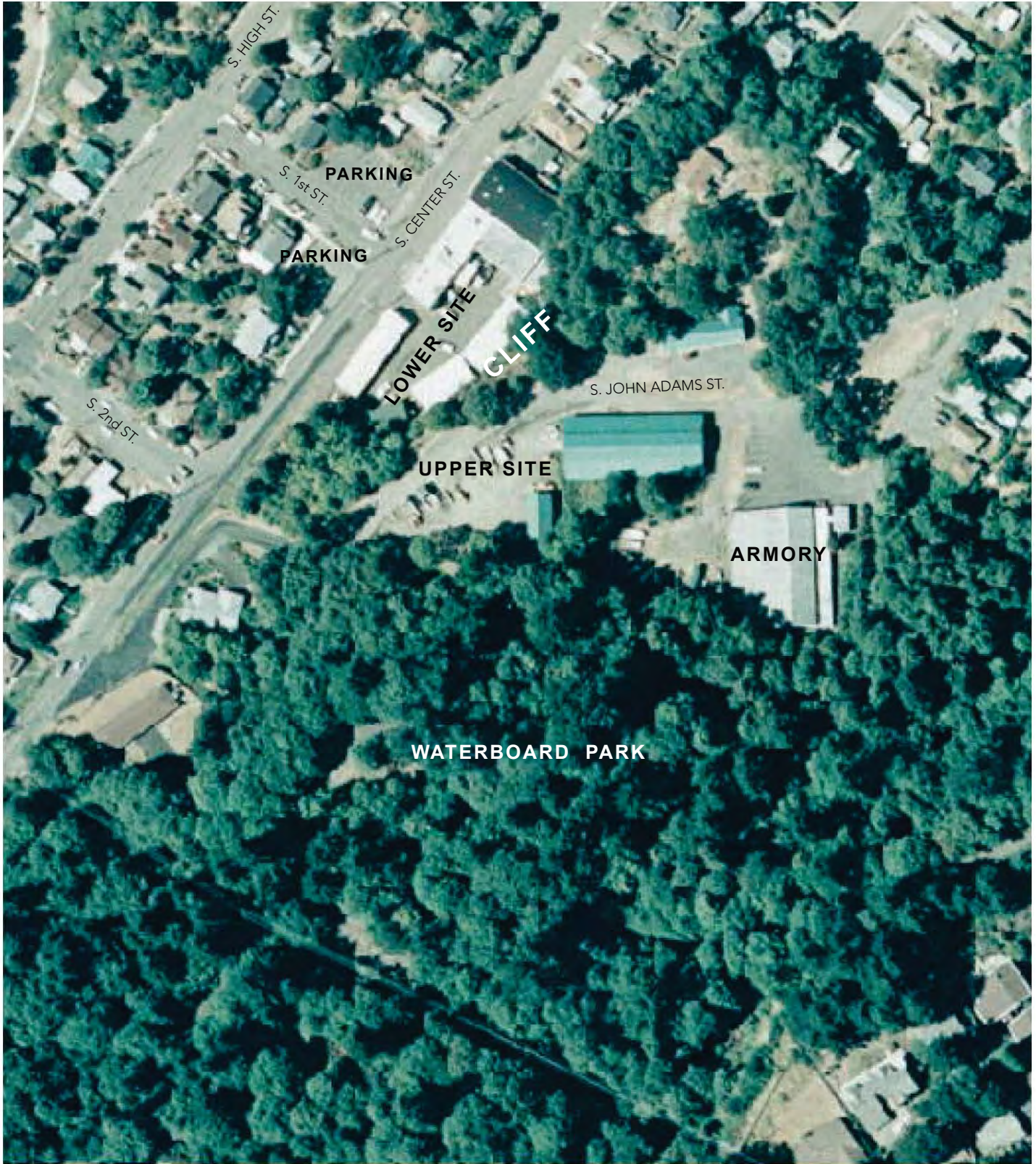
AERIAL OF EXISTING PUBLIC WORKS SITE
