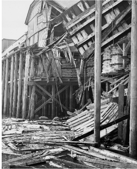
Collision damage from the Aegean Mariner, 1965
