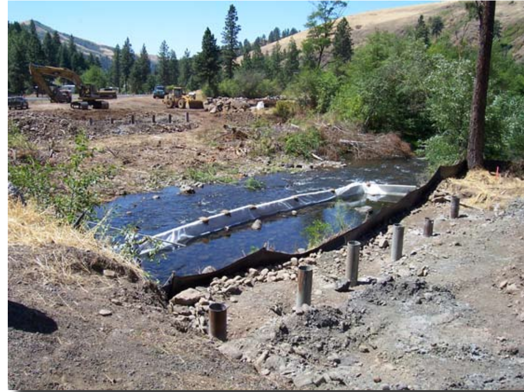
PHOTO 2 - Photo of a similar work area isolation structure on the Umatilla River.
