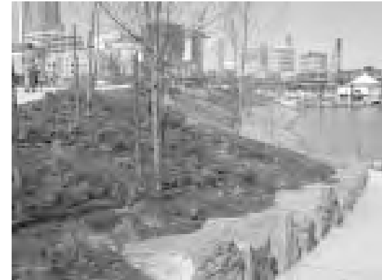
In order to improve habitat along the Willamette River, the City incorporated erosion-control measures as well as native plants into the bank design of the South Waterfront Park addition.
