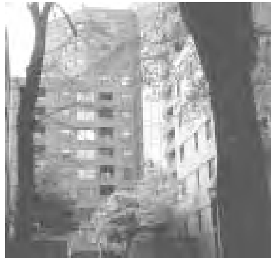
The South Park Square Apartment complex contains a variety of retail stores.
