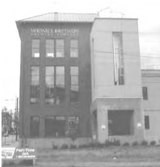
Widmer Brothers Brewery is listed in the National Register of Historic Buildings.
