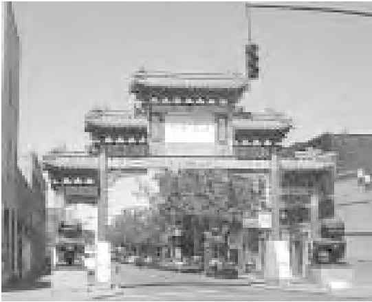
The elaborate Chinatown arch heralds the entrance to the Chinatown/New Japantown Historic District.
