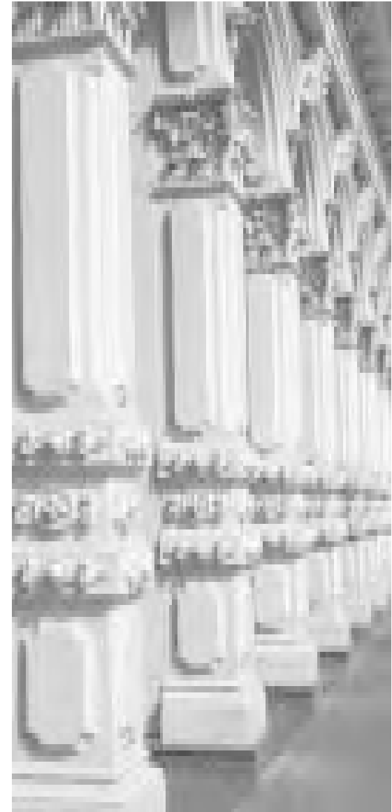
This restored cast iron colonnade was once part of the Ladd and Tilton Bank.
