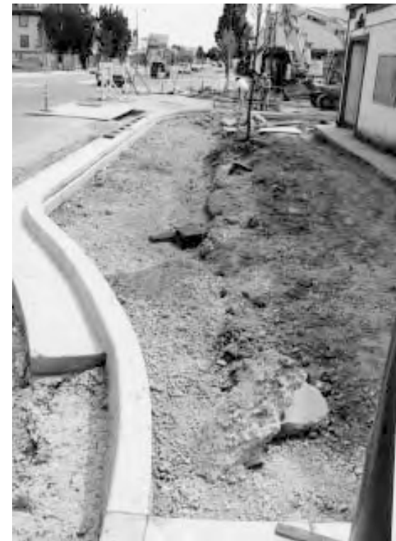
Curb extensions are being installed at certain intersections on MLK.
