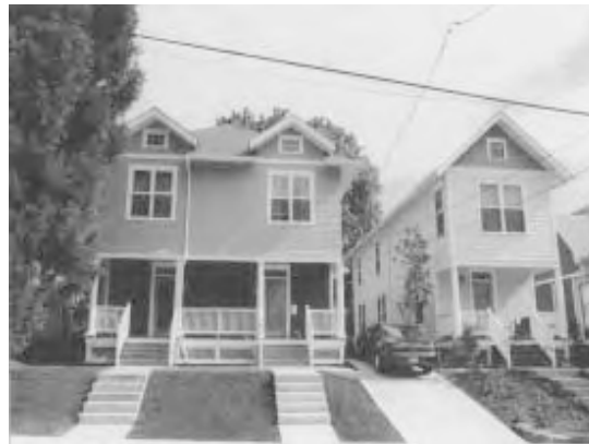
New rowhouses in the Eliot Neighborhood blend in well with the existing housing constructed at the turn of the century.
