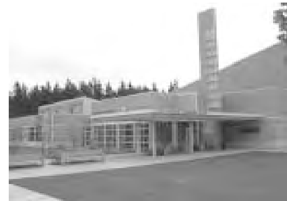
Completed in 1998, the East Portland Community Center adds to the increasing variety of activities along 106 th Avenue.
