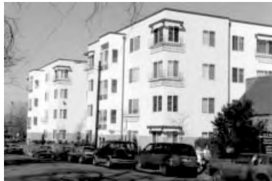
The Dawson Park Apartments are located on N Morris and Vancouver Avenue. This is a high density multifamily use on a street with good bus service close to Emanuel Hospital and employers in the Lloyd Center.
