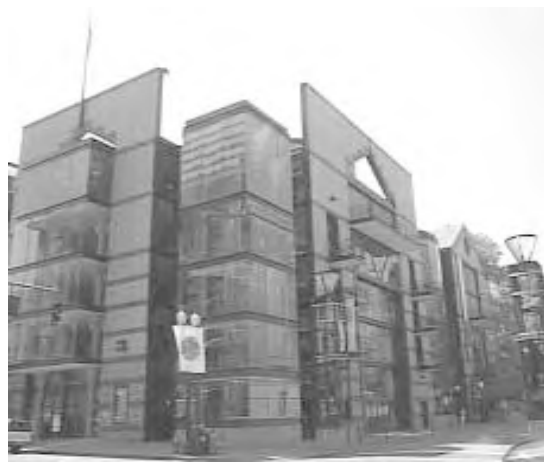
The Performing Arts Center includes three theaters of varying sizes within its main structure.
