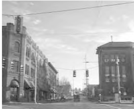
The Russell Street Conservation District is part of the Eliot neighborhood.
