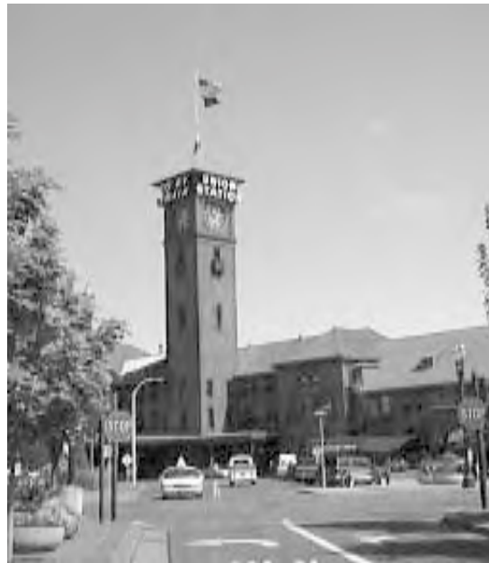
Union Station, above, and the Greyhound Bus Terminal, below right, form the heart of the intermodal transportation center.
