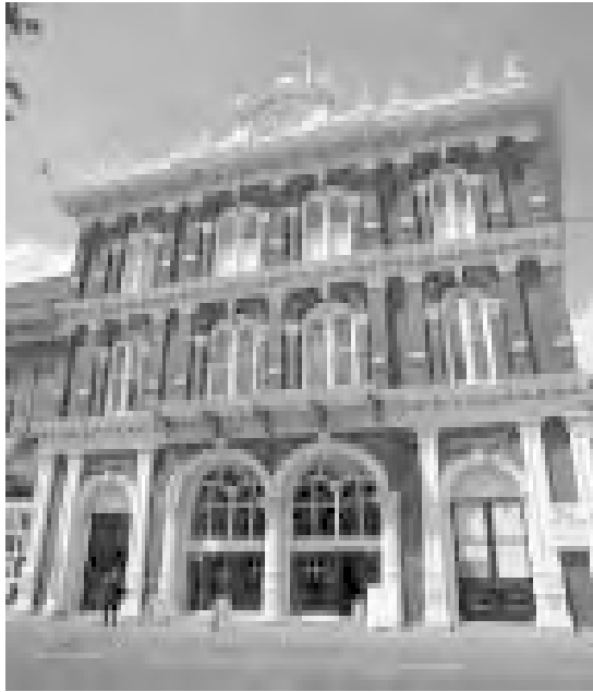
The New Market Block, restored in 1983, contains retail stores, restaurants, and offices.
