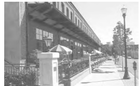
These renovated Hoyt Street railyard warehouse buildings are now new townhouses in the Pearl District.
