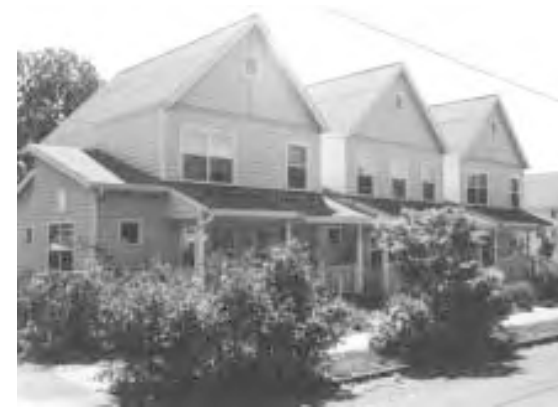
This rowhouse project at NE 6 th Avenue and NE Going won the American Institute of Architect's Essential Housing design competition for this site in 1991.
