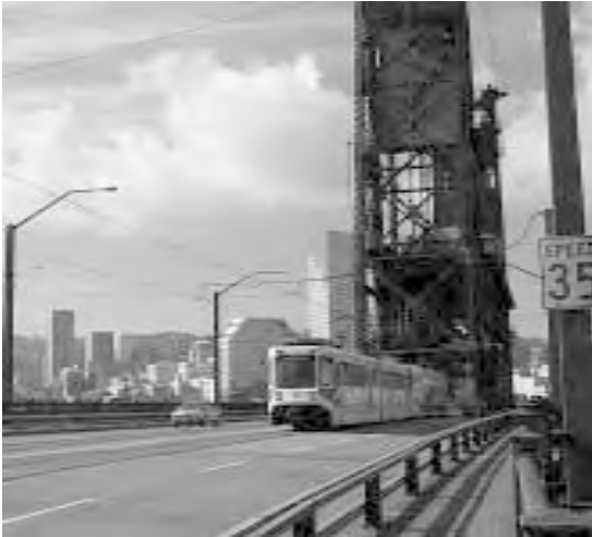
MAX crosses the Steel Bridge toward Downtown on its route from Gresham.
