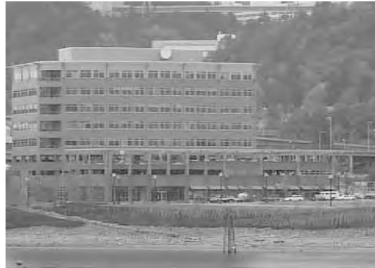
The PG&E Transmission Building at RiverPlace is an energy efficient demonstration project.
