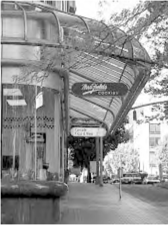
Awning along the PacWest Building
