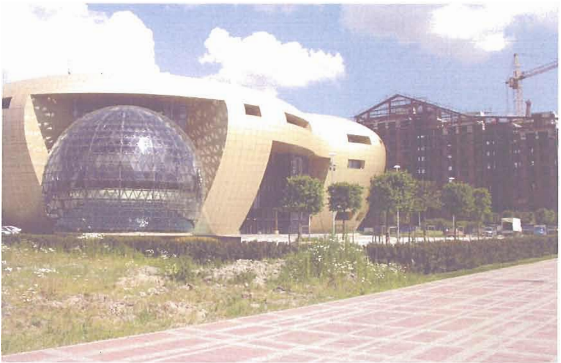
Illustration 4.1. The Baltic Pearl business center, with units under construction.
