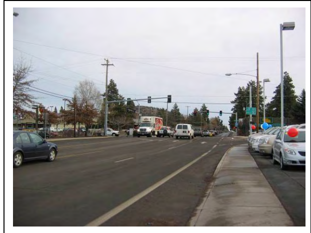
Franklin Avenue @ 3 rd Street: Looking east through intersection from southwest corner. bend 004.jpg
