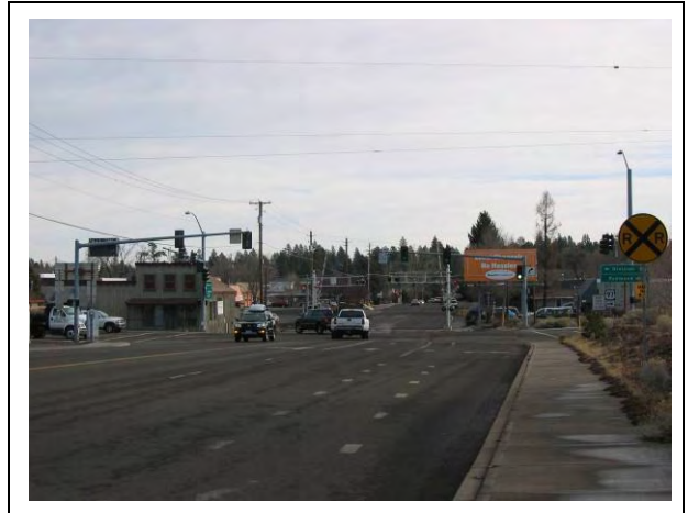
Revere Avenue @ Parkway NB Ramp: Looking east through intersection from south side of Revere Avenue. bend 094.jpg
