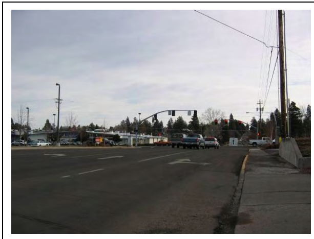
Revere Avenue @ 3 rd Street: Looking east through intersection from south side of Revere Avenue. bend 089.jpg
