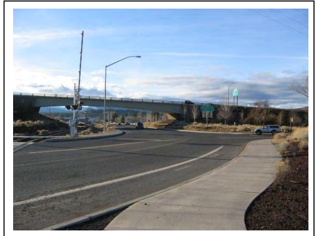
Colorado Avenue @ Parkway NB Ramp: Looking west through intersection from northwest corner. bend 043.jpg
