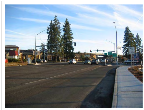
Butler Market Road @ US 97/20: Looking south through intersection from northwest side of US 97/20. bend 071.jpg
