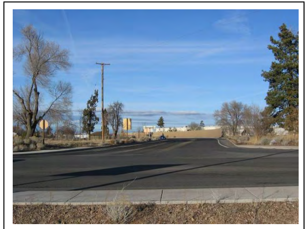
Colorado Avenue @ Parkway NB Ramp: Looking north through intersection from south side of Colorado Avenue. bend 042.jpg
