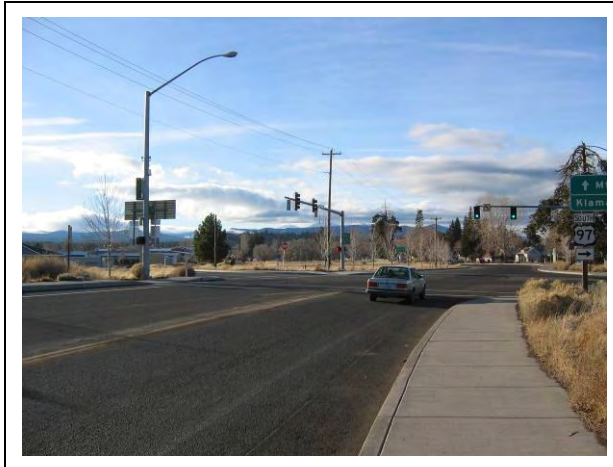
Colorado Avenue @ Parkway SB Ramp: Looking west into intersection from north side of Colorado Avenue. bend 039.jpg
