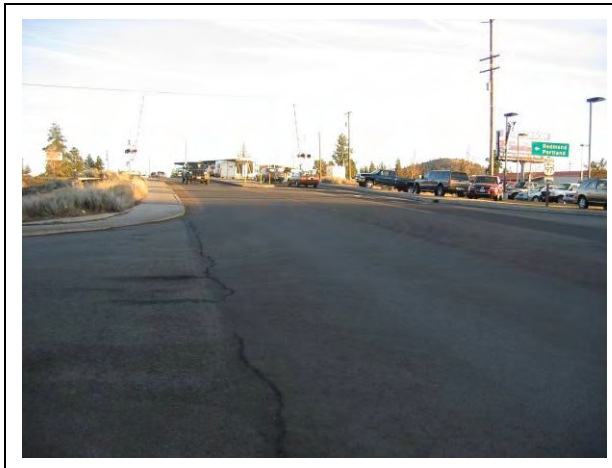
Butler Market Road @ Parkway NB Ramp: Looking east through intersection from the northwest corner. bend 063.jpg
