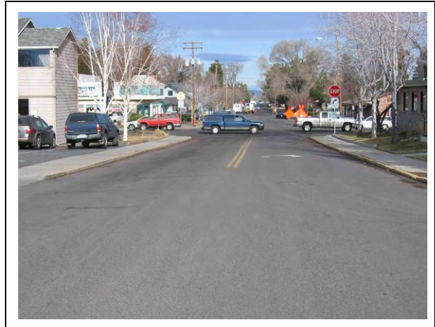
Greenwood Avenue @ 4 th Street: Looking north through intersection from the south. bend 021.jpg
