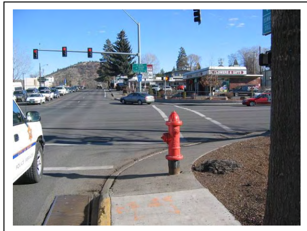
Greenwood Avenue @ 3 rd Street: Sidewalk obstruction looking east along Greenwood Avenue. bend 025.jpg
