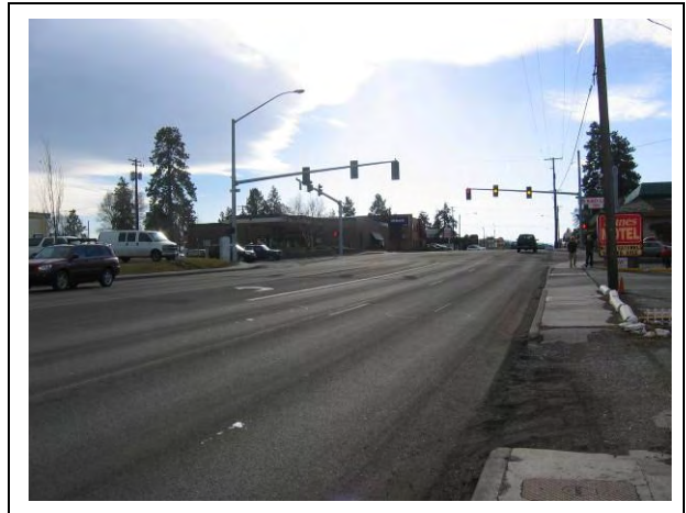
Olney Avenue @ 3 rd Street: Looking south through intersection from northwest side of 3 rd Street. bend 105.jpg
