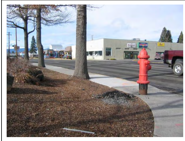
Greenwood Avenue @ 3 rd Street: Side walk obstruction looking west along Greenwood Avenue. bend 026.jpg
