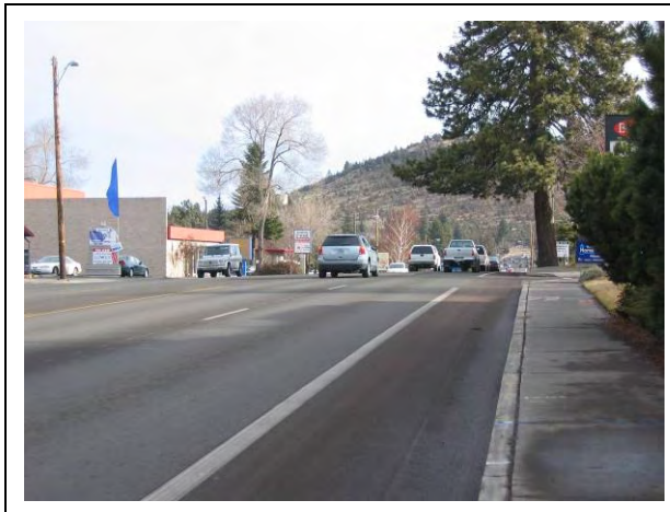
Greenwood Avenue @ 4 th Street: Looking east through intersection along south side of Greenwood Avenue bend 022.jpg
