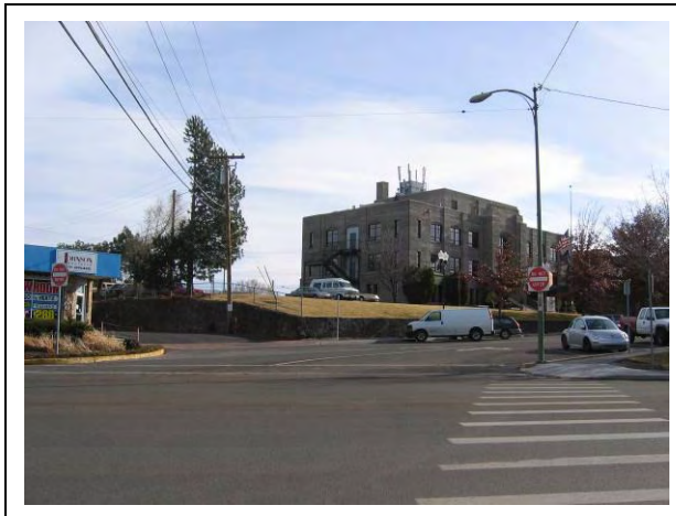
Wall Street @ Bond Avenue: Looking east through intersection from pedestrian crossing. bend 125.jpg
