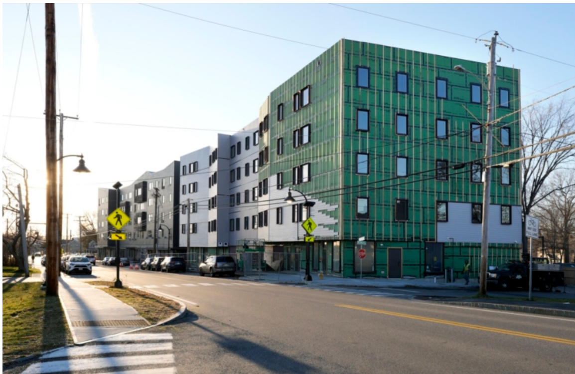
Figure 3.10: West End Apartments in South Portland, ME. (Photo: Brianna Soukup/Staff Photographer, www.pressherald.com , 2023)
