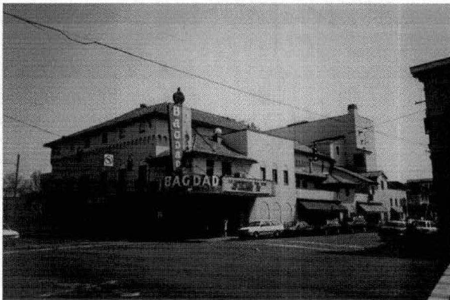
Figure 60. Exterior of the Bagdad Theater, Portland. Photo by Author, April 1998.
