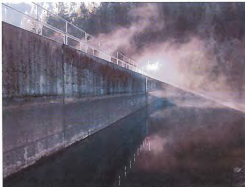
Reservoir and upstream face of dam
