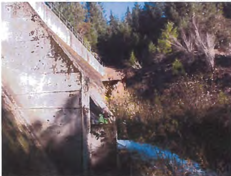
Left abutment and discharge from primary conduit
