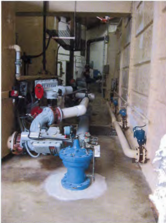
FIGURE 5.3.10 FILTER PIPING
