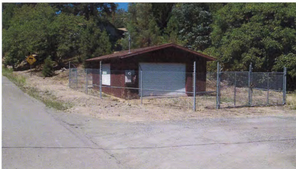
FIGURE 5.5.2 HILL PUMP STATION
