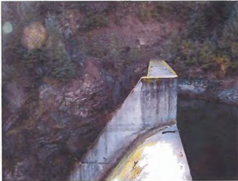
Right side of spillway and right abutment
