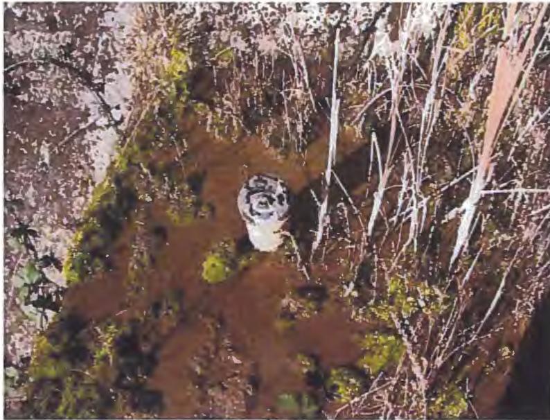
Piezometer at toe next to left abutment
