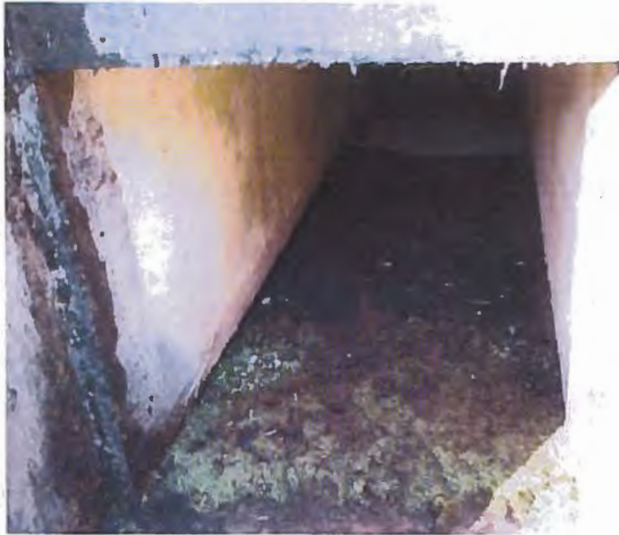
Outlet tunnel for sluice gate
