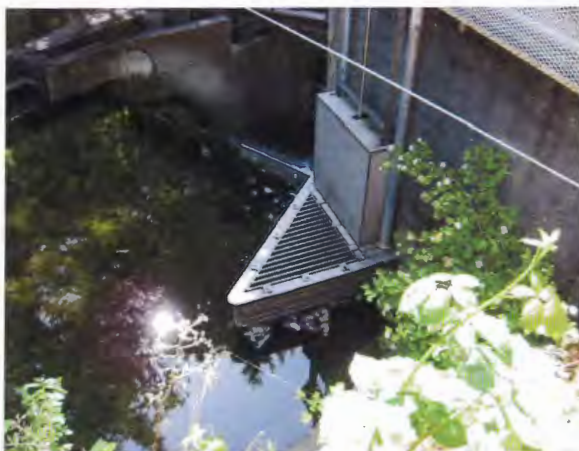
FIGURE 5.2.3 INTAKE SCREEN
