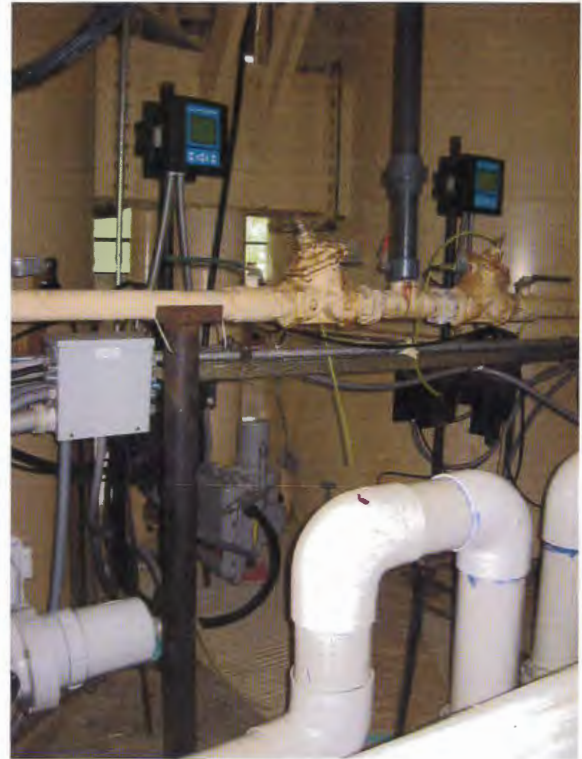
FIGURE 5.3.11 TURBIDIMETERS
