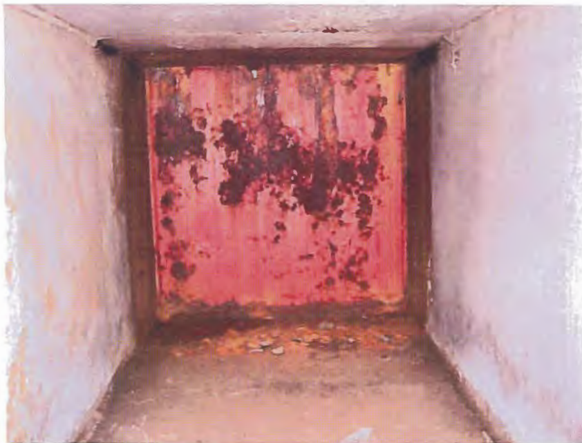
Sluice gate from inside of tunnel
