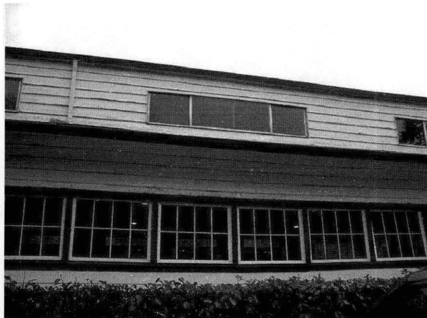
Figure 4.10: Aluminum (clearstory) and Vinyl Window replacements, February 2005.
