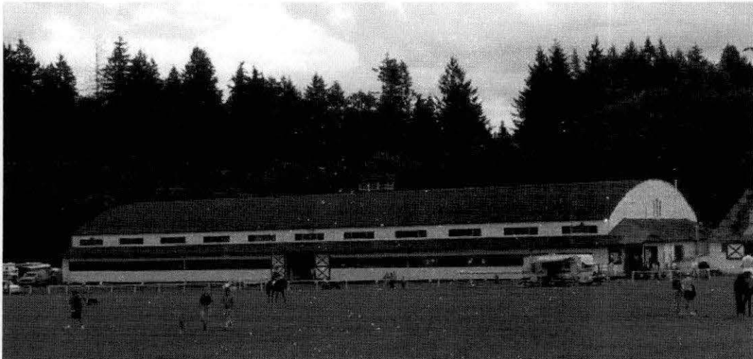
Figure 4.1: Looking south at the arena space and polo field, 2001. (Photo courtesy of the Lake Oswego Hunt)
