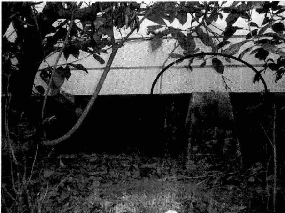
Figure 4.11: Pier on post foundation, February 2005.
