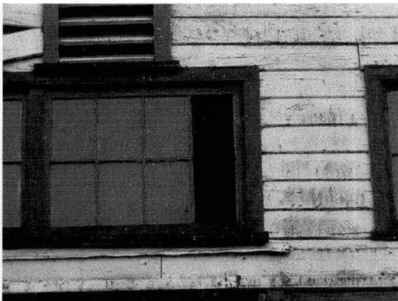
Figure 4.5: Detail view of east façade historic wood windows and vertical vents, November 2004.
