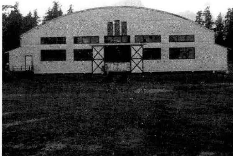
Figure 4.4: East façade historic wood windows and vertical vents, November 2004.
