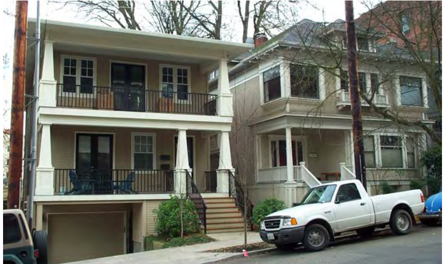
Duplex (2003) to left, shared basement parking facilitated its development on a small urban lot.
