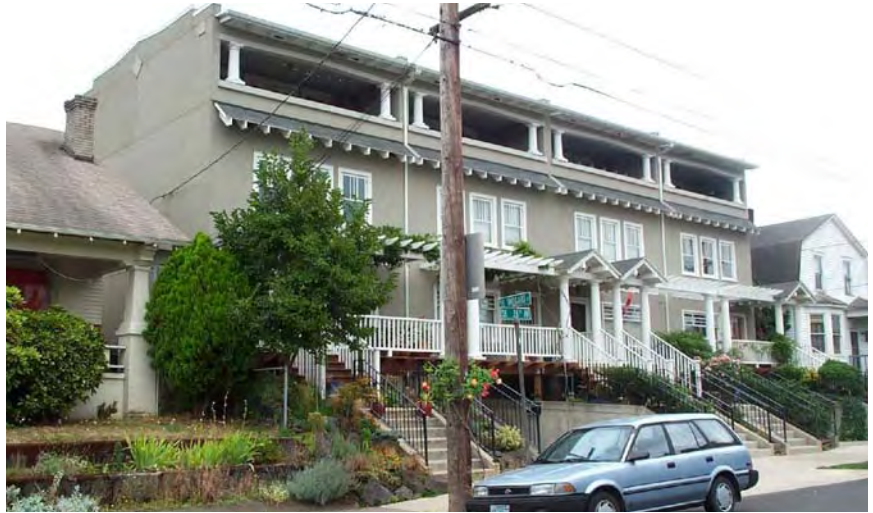
Rowhouses with upper-levels set back within covered terraces, helping to mitigate their four-level height.
