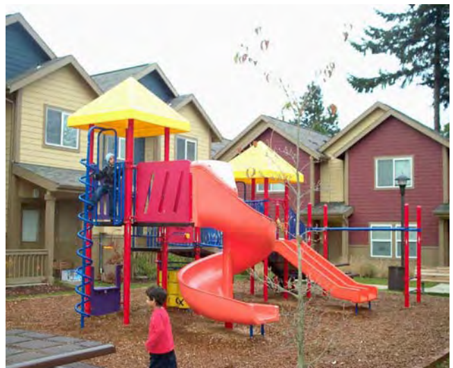
Courtyards are especially useful in providing space of sufficient size to be usable by children, particularly when it is not possible to provide private yards large enough to serve as play space.
