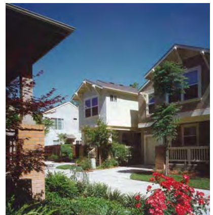
Metro Square, Sacramento, CA (Mogavero Notestine Associates). 12'-wide accessway reads either as a wide walkway or a narrow drive
