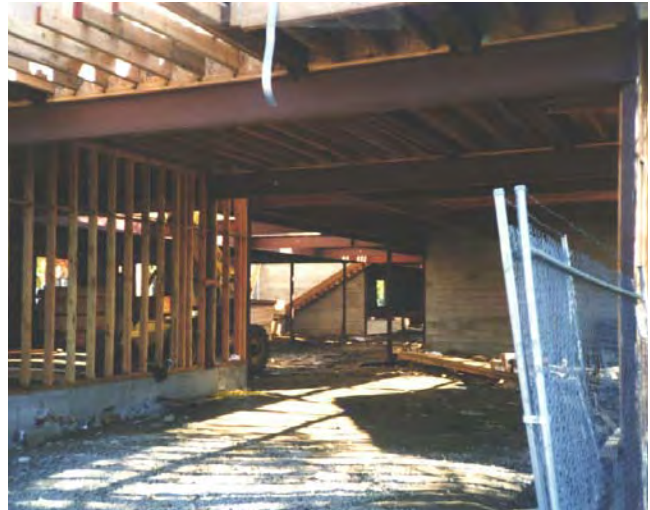
A combination of concrete block, steel, and wood framing can now be used as long as the parking is solely for the residents. Builders are often more familiar with steel and wood frame methods of construction.
