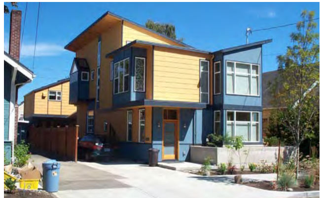
Secondary unit, over garage, allowed this house to meet R2 density requirements
