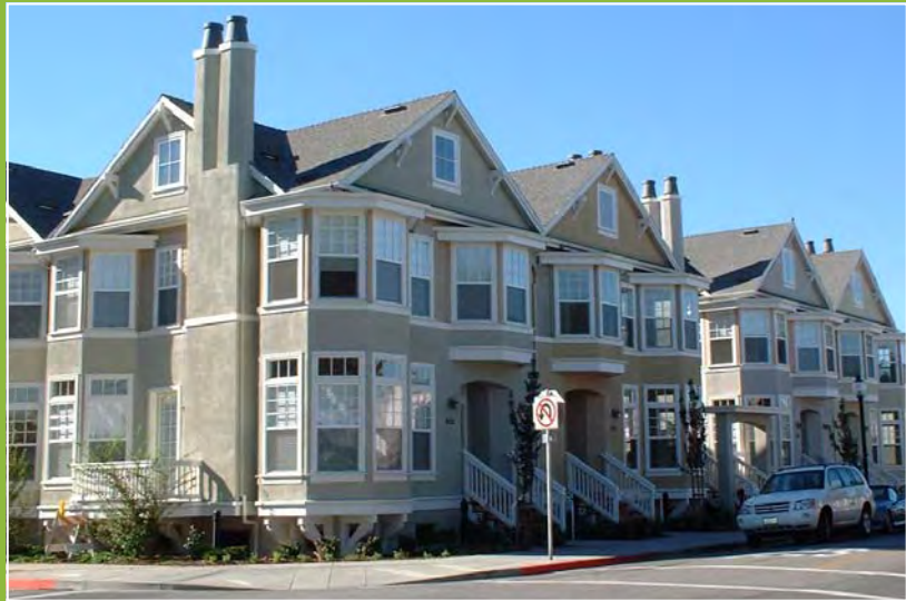
Developers of medium density infill projects are looking at shared structured parking as a viable strategy to increase density while providing usable open space and meeting parking demand.
