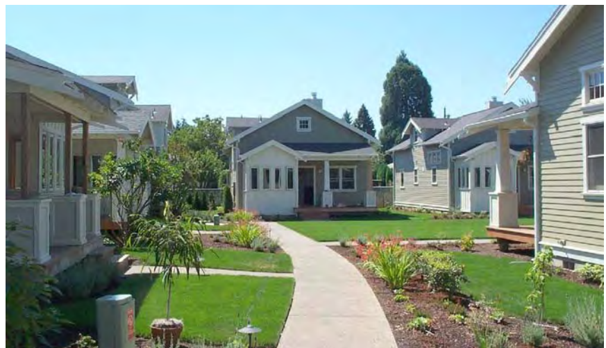
Recent Portland courtyard housing project, “Hastings Green,” featuring cottages oriented to a shared courtyard. Developed as condominiums, all units sold before project completion, indicating market demand for such housing.
