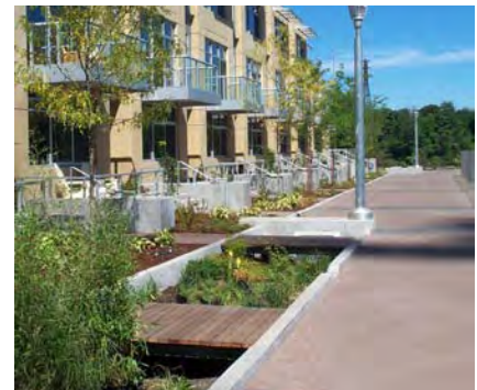
Stormwater planters integrated into the design of shared pedestrian/vehicle space (Meriwether Townhouses)
