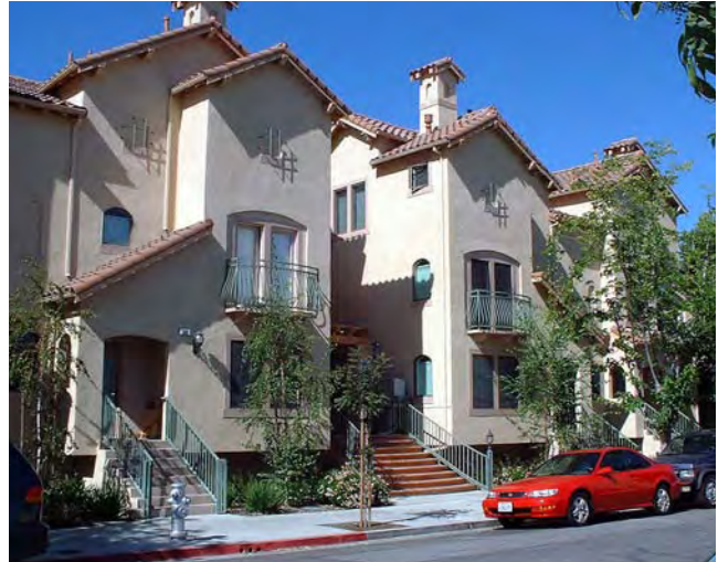
Sub-grade parking is seen in many new developments because it places parking underneath buildings, allowing the site to support more building area and open space.
