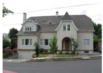
SE 32nd & Pine (1926). Example of a classic Portland corner duplex. Designed to provide the appearance of a single-family house, with two units within a single house-like mass and entrances facing separate streets.
