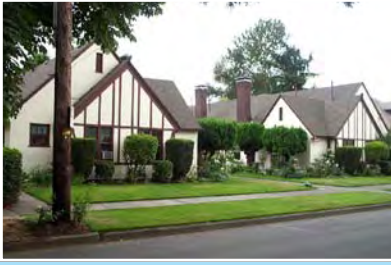
Courtyard apartments NE Multnomah & 22nd (1927)
