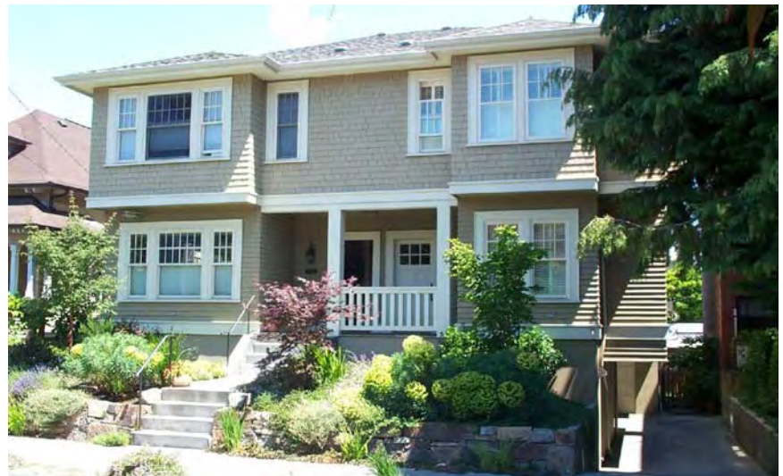
Four-unit townhouse cluster in Seattle, with partially-excavated garages.
