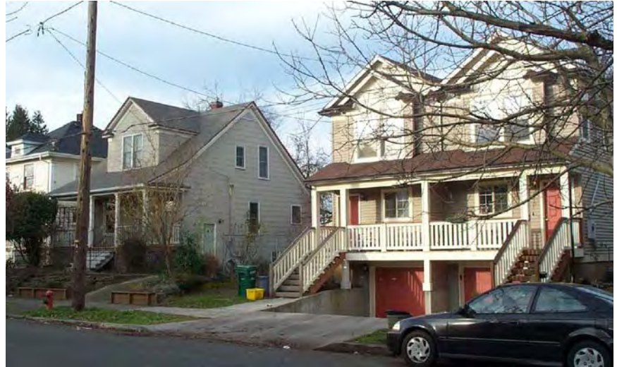
Rowhouses with excavated lower-level garages
