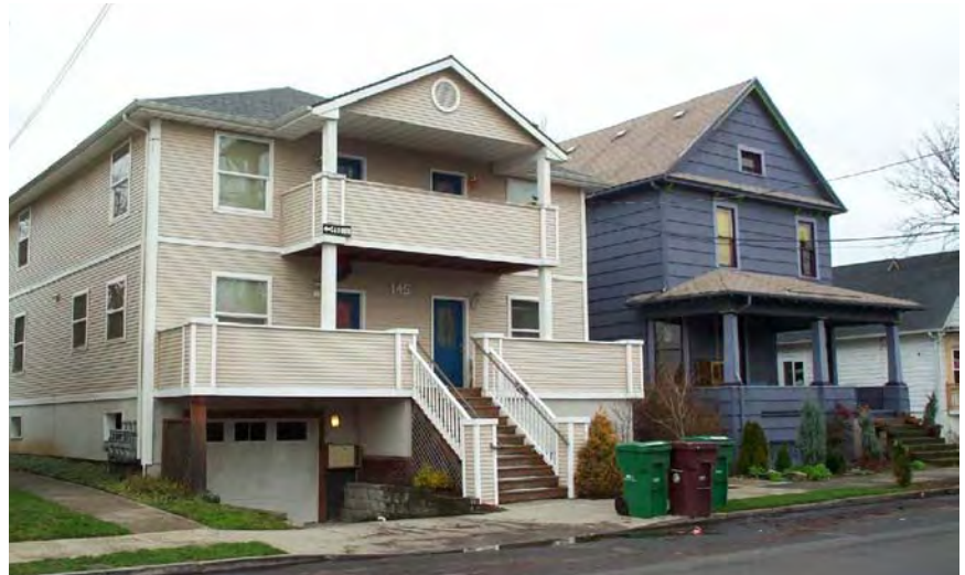
Fourplex with excavated basement parking
