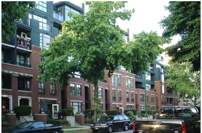
Upper-level step backs, differing façade materials and darker colors help focus attention on bottom two-three levels, de-emphasizing the presence of the upper stories. (Vancouver, BC)
