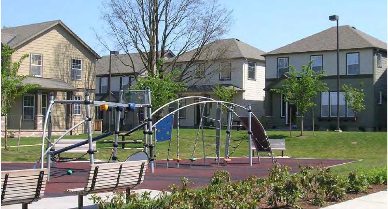
Detached houses fronting a common green with play equipment (R2 zone, New Columbia).
