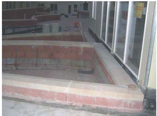
Waterproofing and flashing protects the building and podium around integrated planters
