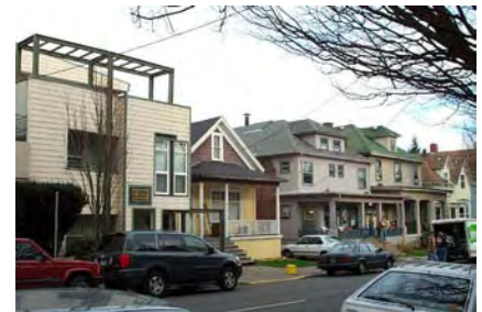
Contemporary infill continues street frontage rhythm
