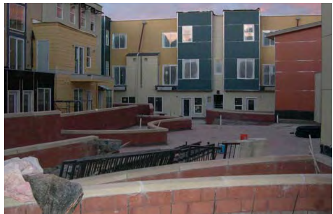
A parking podium in Boulder, CO with integrated planters under construction.
