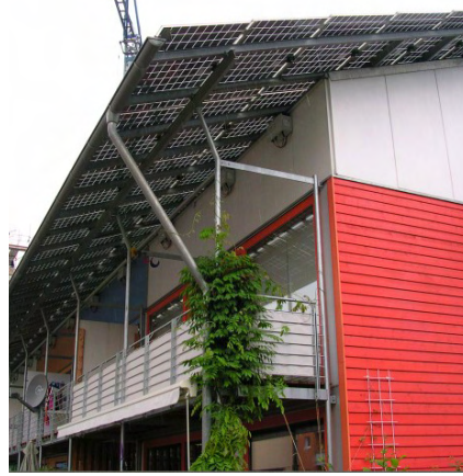
Vauban District, Germany. A former military base was redeveloped into an environmentally-sustainable community of family housing. These buildings integrate vernacular forms with green features. Pitched roofs with overhanging eaves serve as platforms for solar panels; an arrangement which could be at home with Portland's building traditions.
