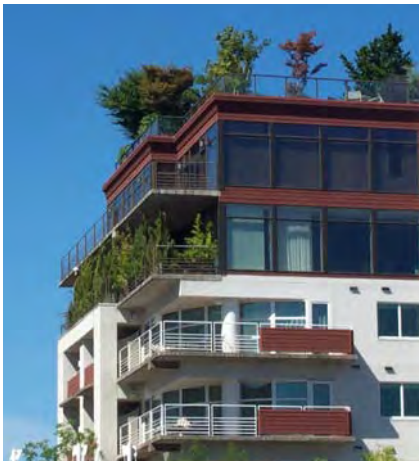
The predominance of glass, combined with the subdued colors, step backs and terrace plantings of upper levels diminish apparent building scale.
