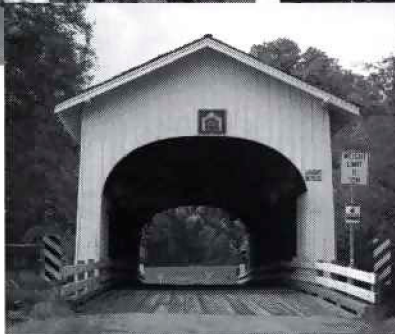
Harris Covered Bridge
