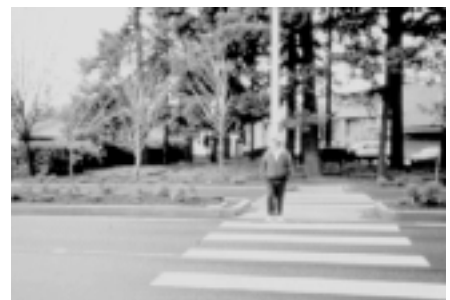
Median refuge island allow pedestrians to cross one direction of vehicle travel at a time.
