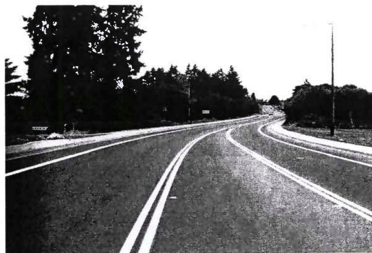
Looking East Along SW Farmington Road At Church Driveway
