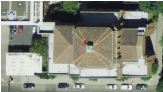
Aerial view - hipped western roof, central dome, eastern gabled roof
