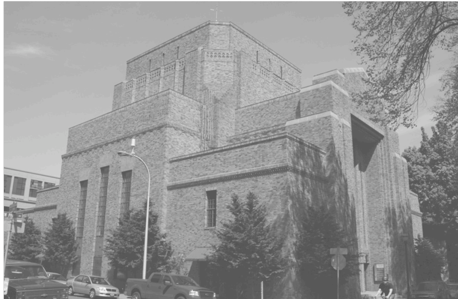
Three-quarter view of southeast corner
