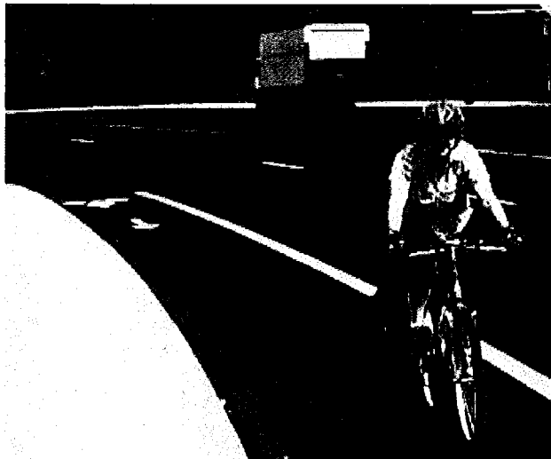
Bicycle lanes on busy Kane Drive connect cyclists safely to the 40-Mile Loop.
