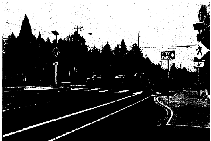
Raised medians benefit pedestrians by allowing them to cross only one direction of traffic at a time.
