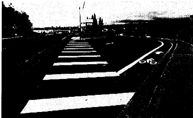
Freight improvements at NE 181st Avenue and Wilkes Road allow easier access to Interstate 84.
