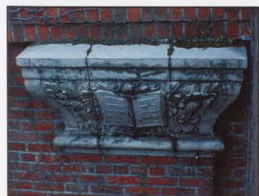
FIGURE 13: TERRA COTTA PILASTER CAPITAL
