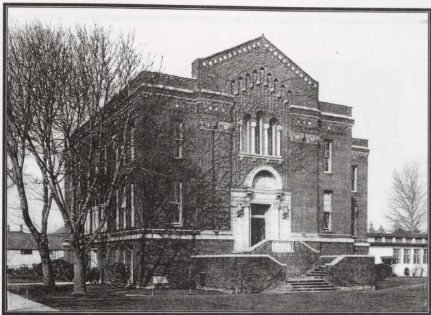
FIGURE 117: EDUCATION BUILDING SOUTHEAST ELEVATION – CIRCA. 1935 Lawrence Collection, Courtesy of Special Collections, Knight Library, University of Oregon.
