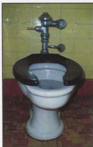
FIGURE 48: ORIGINAL TOILET FIXTURE
