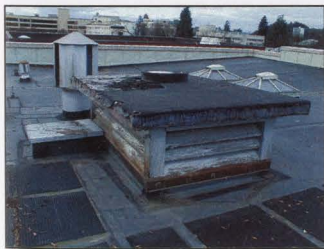
FIGURE 32: HISTORIC ROOF VENT "PENTHOUSE"
