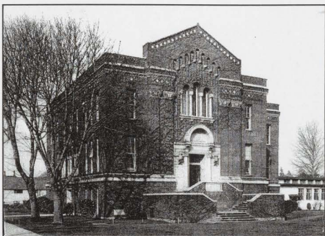
FIGURE 1: 1916 EDUCATION BUILDING SOUTHEAST ELEVATION – CIRCA. 1935 Lawrence Collection, Courtesy of Special Collections, Knight Library, University of Oregon.
