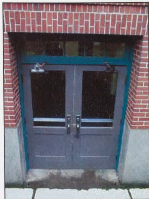
FIGURE 76: FIRST FLOOR ENTRY DOORS AT SOUTH ELEVATION
