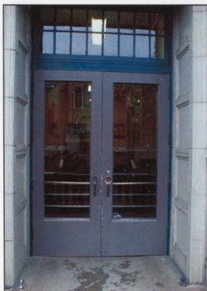
FIGURE 38: PAIRED DOORS WITH \frac{1}{2} " LENGTH LIGHT AND TRANSOM AT MAIN ENTRY.
