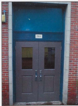
FIGURE 39: PAIRED SOLID WOOD DOORS AT SOUTH ENTRY WITH TRANSOM REMOVED.
