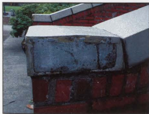
FIGURE 18: ALTERATION OF TERRA COTTA COPING, 1951
