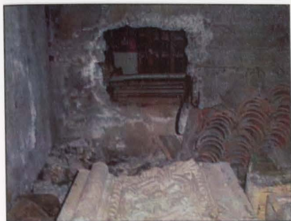
FIGURE 102: STAIR VAULT Hidden access to the stair vault of the Education Building was found off the mechanical room, 112. The terra cotta was found in this space. A pilaster capital and a stack of terra cotta roofing tiles are pictured in the foreground.
