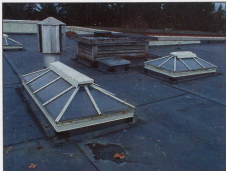
FIGURE 35: GABLED SKYLIGHTS WITH OPERABLE VENT CAPS
