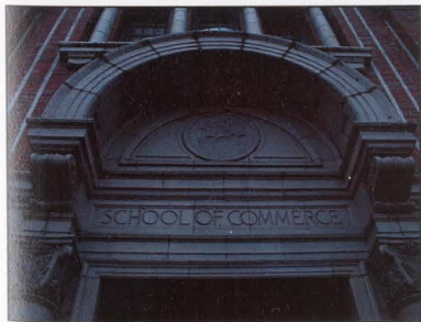
FIGURE 51: DETAIL ABOVE MAIN ENTRY
