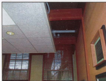
FIGURE 19: SUSPENDED CEILING, RM 201
