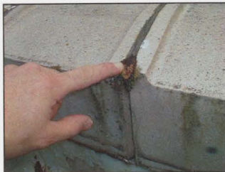
FIGURE 72: LATEX SEALANT BETWEEN PARAPET COPING
