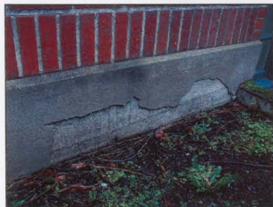
FIGURE 21: STUCCO DETERIORATION
