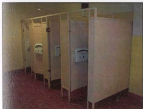
FIGURE 88: ORIGINAL BATHROOM STALLS
