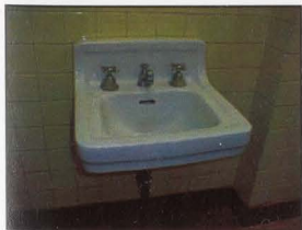
FIGURE 49: ORIGINAL SINK FIXTURE
