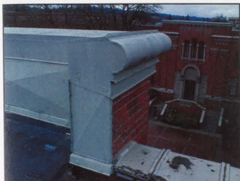
FIGURE 56: BACK OF CAVITY WALL WITH COPPER COPING INSTALLED
