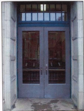
FIGURE 75: MAIN ENTRY DOORS AT WEST ELEVATION
