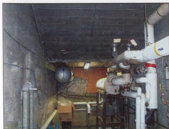
FIGURE 59: FOUNDATION STEM WALL UNDER STAIR VAULT. NOTE THE COLD JOINTS AND THE BOARD FORMED MARKS
