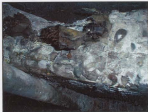
FIGURE 22: EMBEDDED WATER PROOF MEMBRANE
