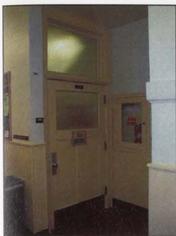
FIGURE 86: ROOM 364. ALL ORIGINAL MILLWORK
