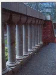
FIGURE 63: MECHANICAL ABRASION OF GLAZE FROM BICYCLE CHAINS
