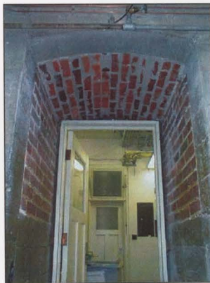
FIGURE 60: SEGMENTAL BRICK ARCH PASSAGE THROUGH THE FOUNDATION WALL TO THE MECHANICAL ROOM
