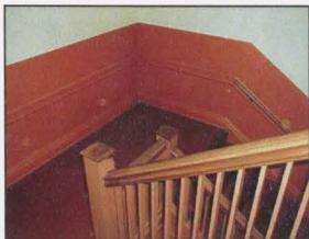
FIGURE 89: STAIRWELL WITH MOLDINGS, RAILS, BALUSTERS AND NEWELS
