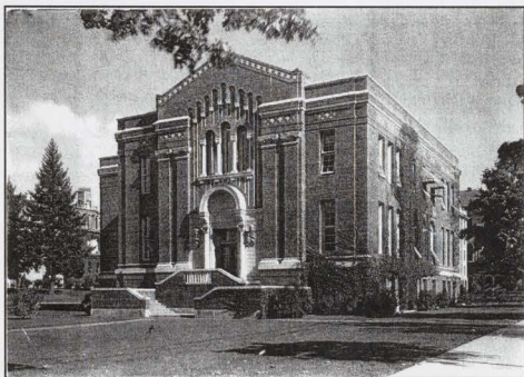
FIGURE 2: 1921 COMMERCE HALL NORTHWEST ELEVATION – CIRCA. 1930 Lawrence Collection, Courtesy of Special Collections, Knight Library, University of Oregon
