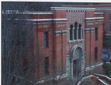
FIGURE 53: WEST SIDE OF THE NORTH ELEVATION – COMMERCE HALL
