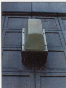
FIGURE 15: HIGH PRESSURE SODIUM LIGHTS REPLACED THE ORNAMENTAL LANTERNS THAT FLANKED THE ENTRY
