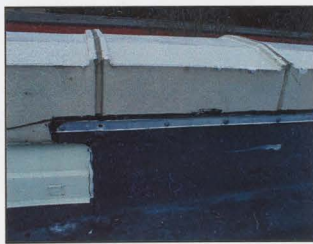
FIGURE 33: LEAD ANCHOR NAILS INSTALLED THROUGH TERRA COTTA COPING TO HOLD THE ROOF MEMBRANE'S RETAINING BAR
