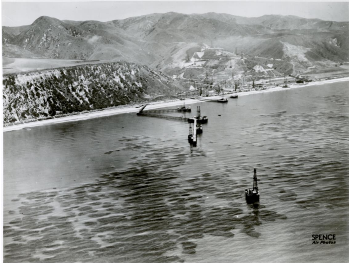
Figure 3.2. Tideland drilling piers extend into the Pacific Ocean at the Rincon Field in Ventura County, California, 1938. Kelp beds are visible in the foreground, which are known to capture and sequester oil. American Petroleum Institute Photograph and Film Collection, Series 1: Historical Photographs, Collection no. 711, Archives Center, National Museum of American History, Smithsonian Institution, Washington, D.C.
