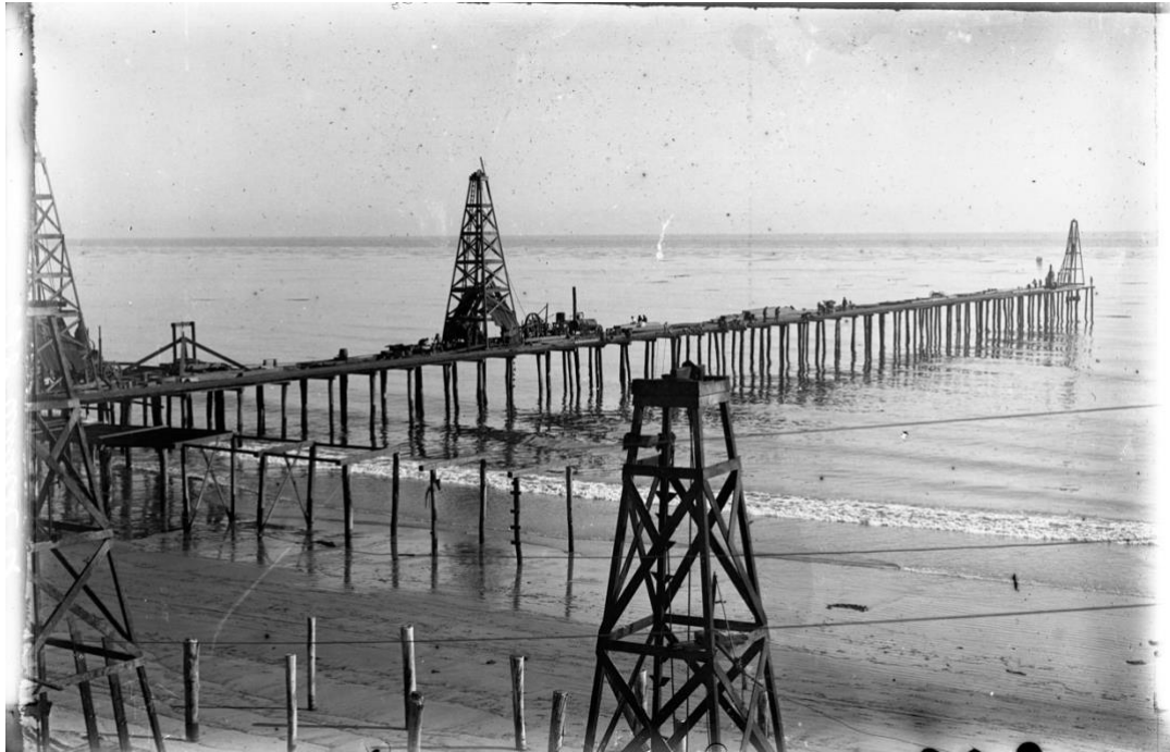
Figure 2.3. John B. Treadwell's pier extends into the sea at Summerland, California. Treadwell abandoned the pier in the early 1900s, but his well casings persisted in the shoreline into the twenty-first century. Photo by Ralph Arnold, ca. 1906, United States Geological Survey, Denver Library Photographic Collection, Denver, Colorado.
