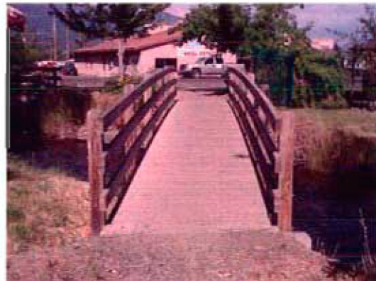
Figure 2-4: Accessway linking N Main Street and E Pine Street.
