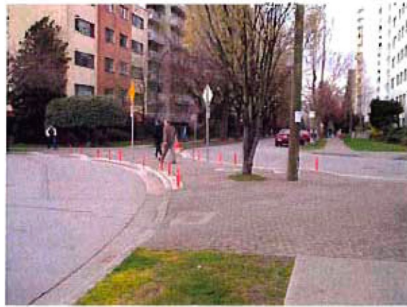
Figure 5-25: Bicycle/pedestrian only refuge island diverts auto traffic.
