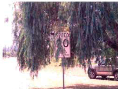
Figure 2-13: Vegetation obstructing a School Speed Zone sign on S College Street.
