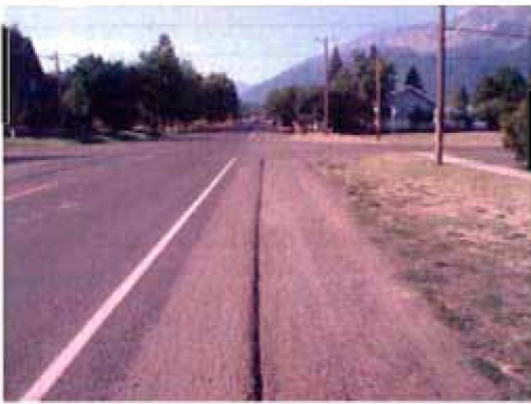
Figure 3-7: S Main Street near Fourth Street (existing conditions).
