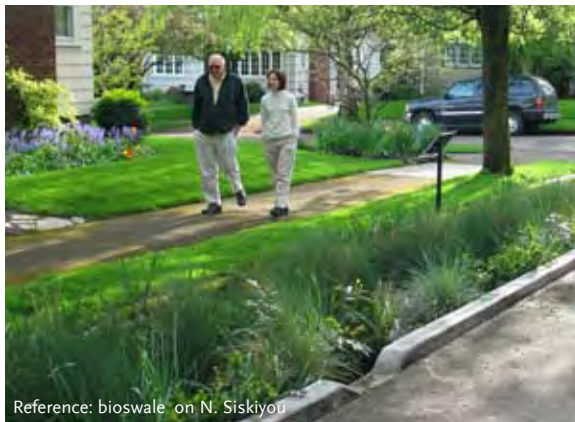
Reference: bioswale on N. Siskiyou
