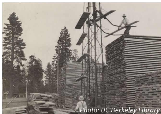
Lumber piling machine at McCloud Lumber, 1920
