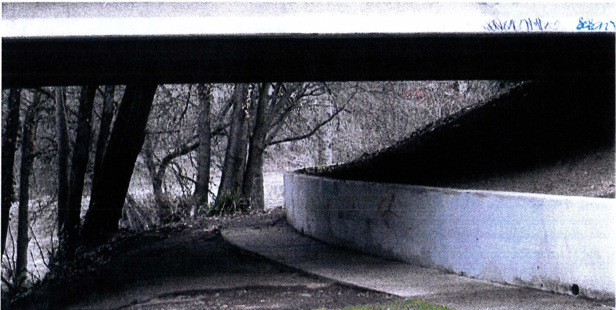
Existing bridge undercrossing conditions
