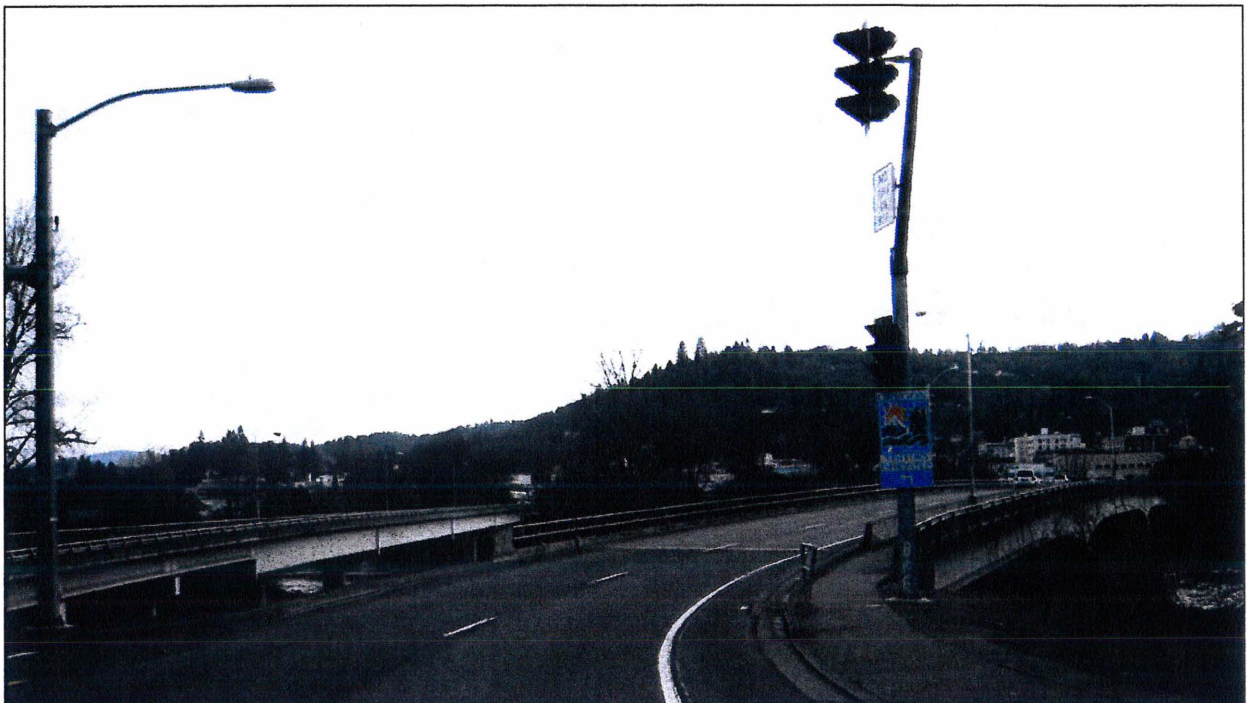
Existing Oak Avenue Bridge looking east
