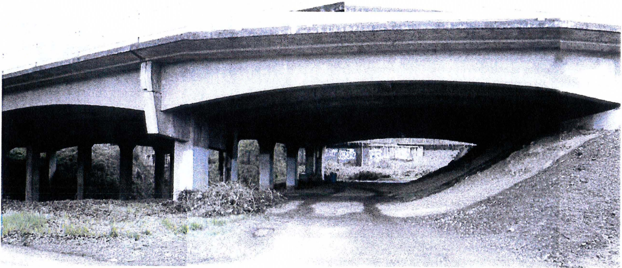
Existing Deer Creek bridge undercrossing
