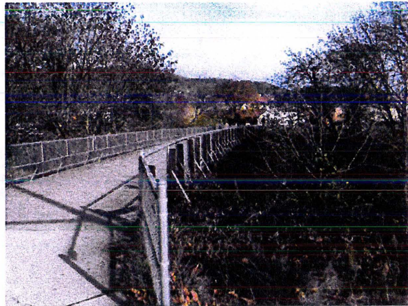
Existing Deer Creek trail on trestle bridge
