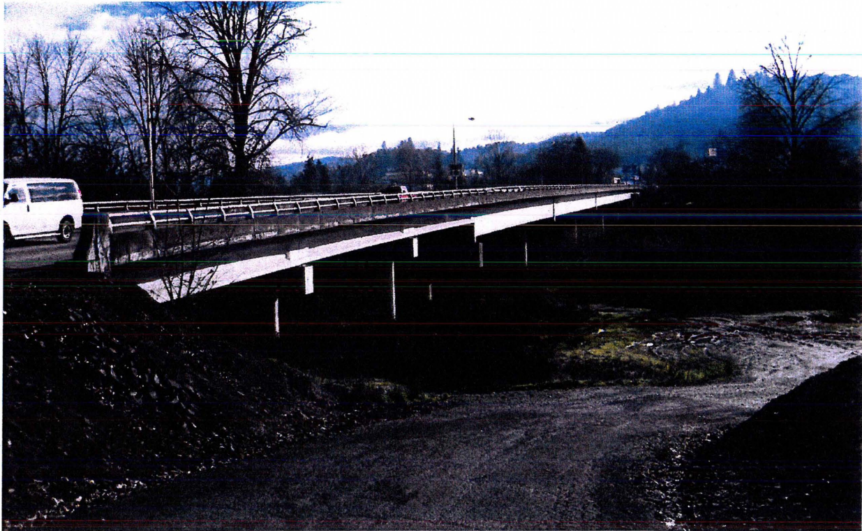
Existing access to private and ODOT property between the Oak and Washington Avenue bridges
