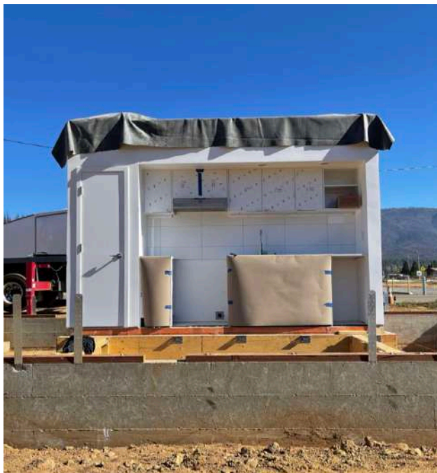
[Left] Image of a prefabricated wet core module Source: atelierjones LLC
