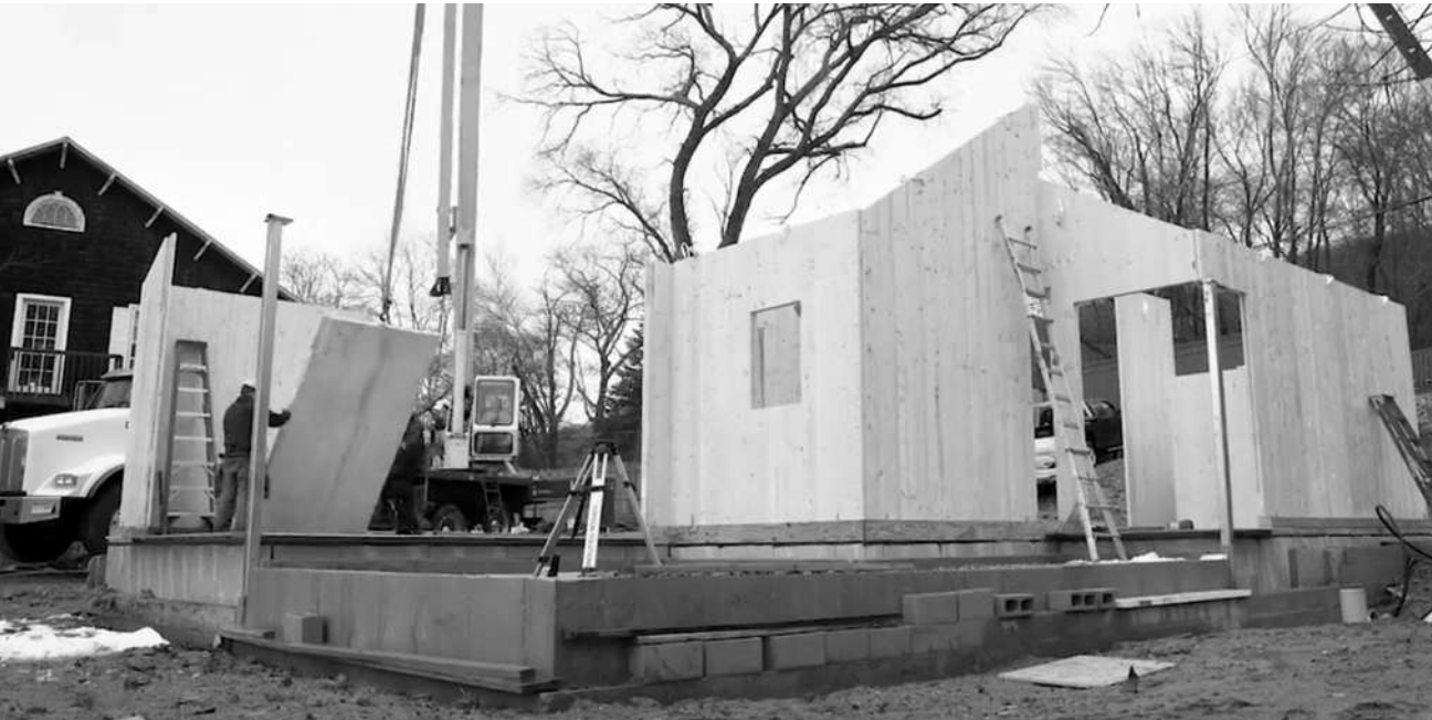
[Top] Pre-designed kit-of-parts modules Source: OPAL / SHELTER
