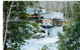
Fallingwater Under Scaffolding
