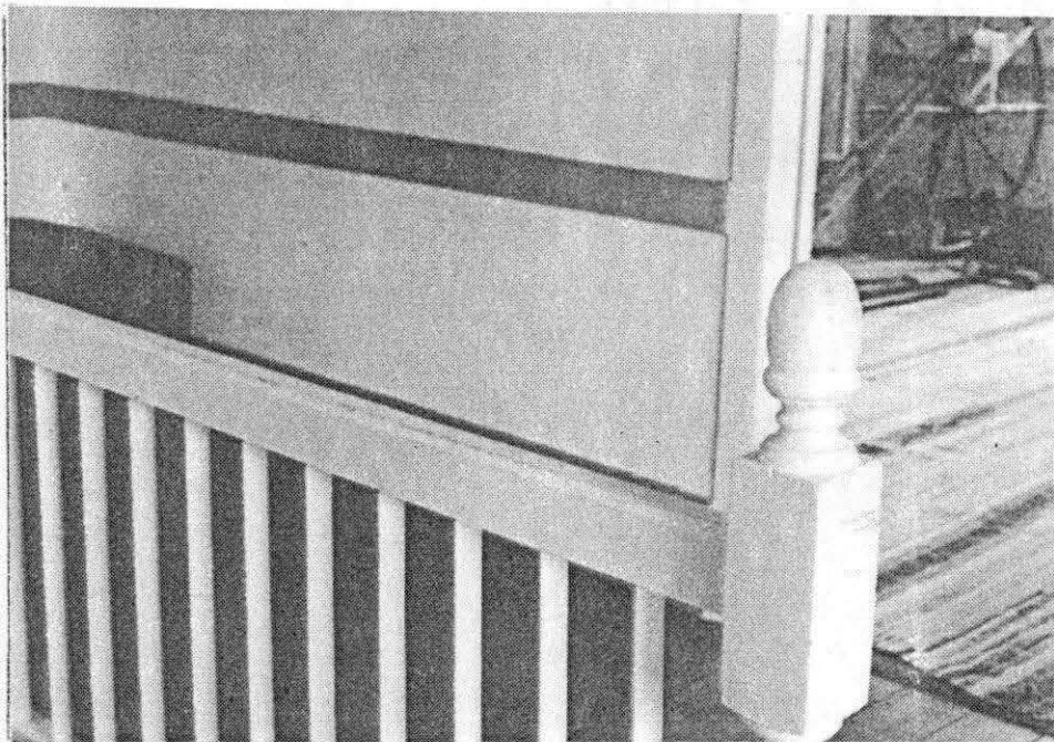
Figure 7. Upstairs hall of Giesy-Kraus house.
