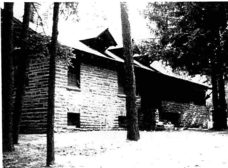
Figure 31. Log infill of windows, north facade, Rocky Point Lodge, Heyburn State Park, 1991.
