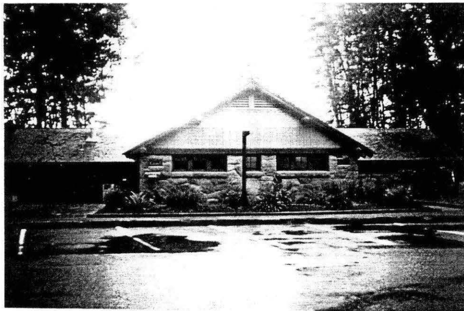
Figure 40. North entrance, concession building, Jessie M. Honeyman Memorial State Park, 1991.
