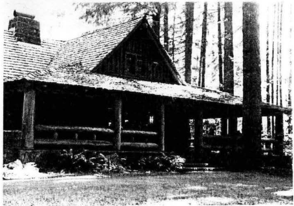
Figure 36. West entrance near concession area, Silver Falls Lodge, Silver Falls State Park, 1991.
