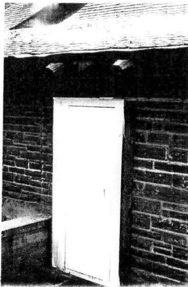
Figure 33. Door to walk-in cooler for kitchen at Rocky Point Lodge, Heyburn State Park, Idaho, 1991.
